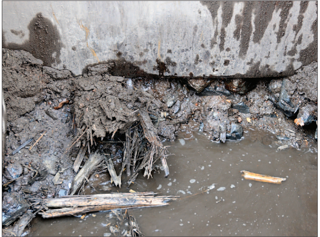
Disturbed timber and cobbles, facing north 13
