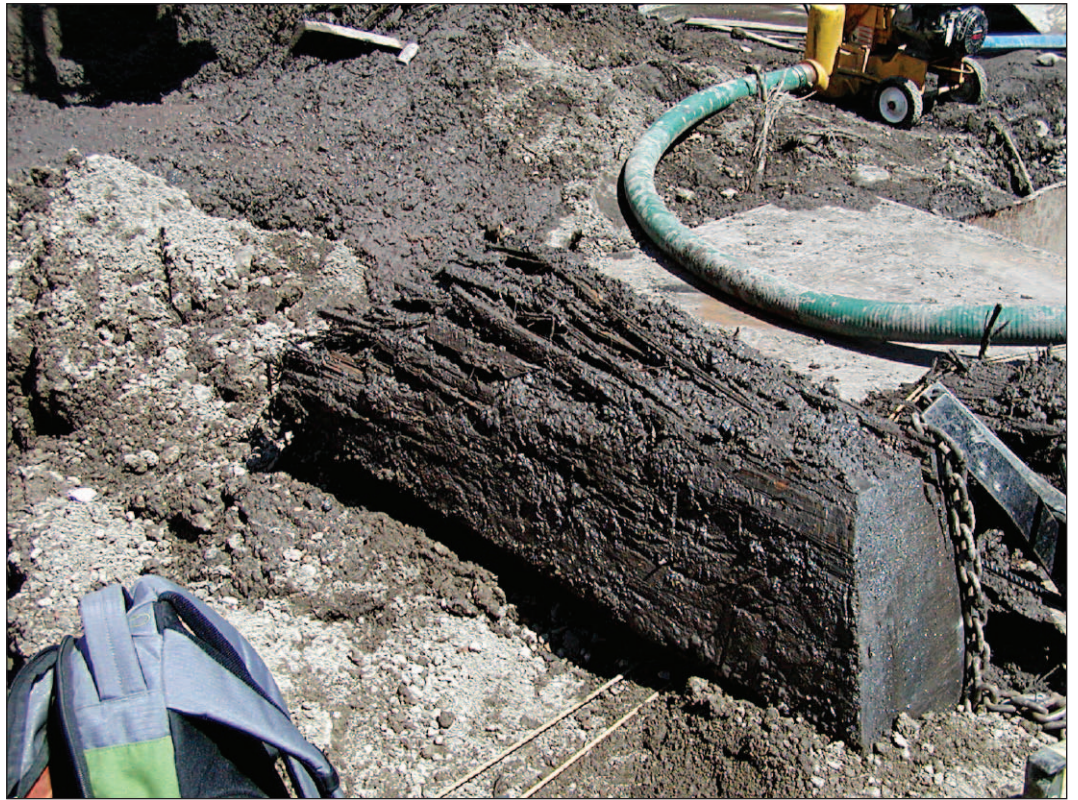
Another removed timber 16
