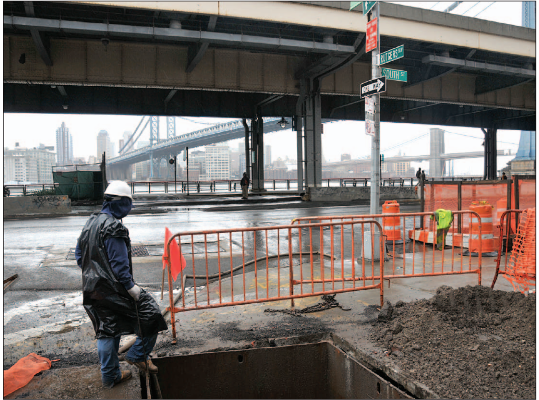
Excavation at Rutgers & South Street, facing south 9
