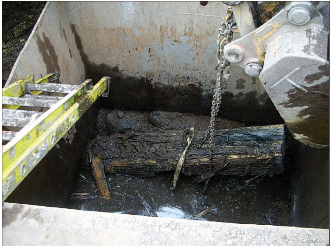
Removal of a timber from the second course 14
