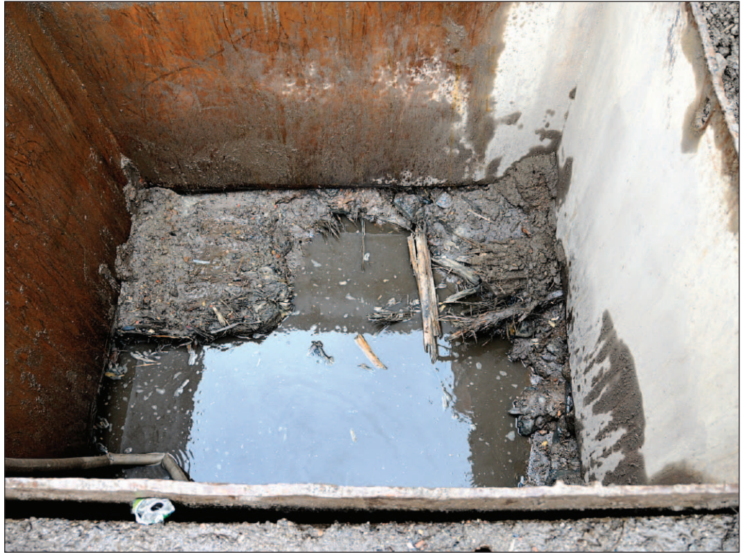
Remains at ~4ft depth facing west 11
