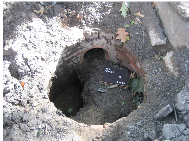
4 D2, a drop inlet, an extant example of the park's 1930s infrastructure. (10/19/09)
