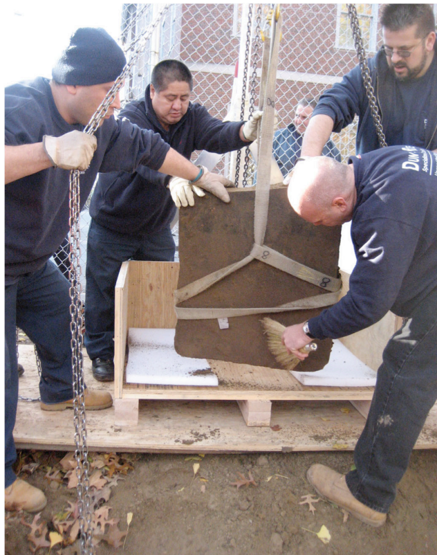
14 The bottom half of the James Jackson headstone being removed by Dun-Rite Art Movers. A gantry was employed to carefully extract both halves of the stone from the ground. (11/16/09)
