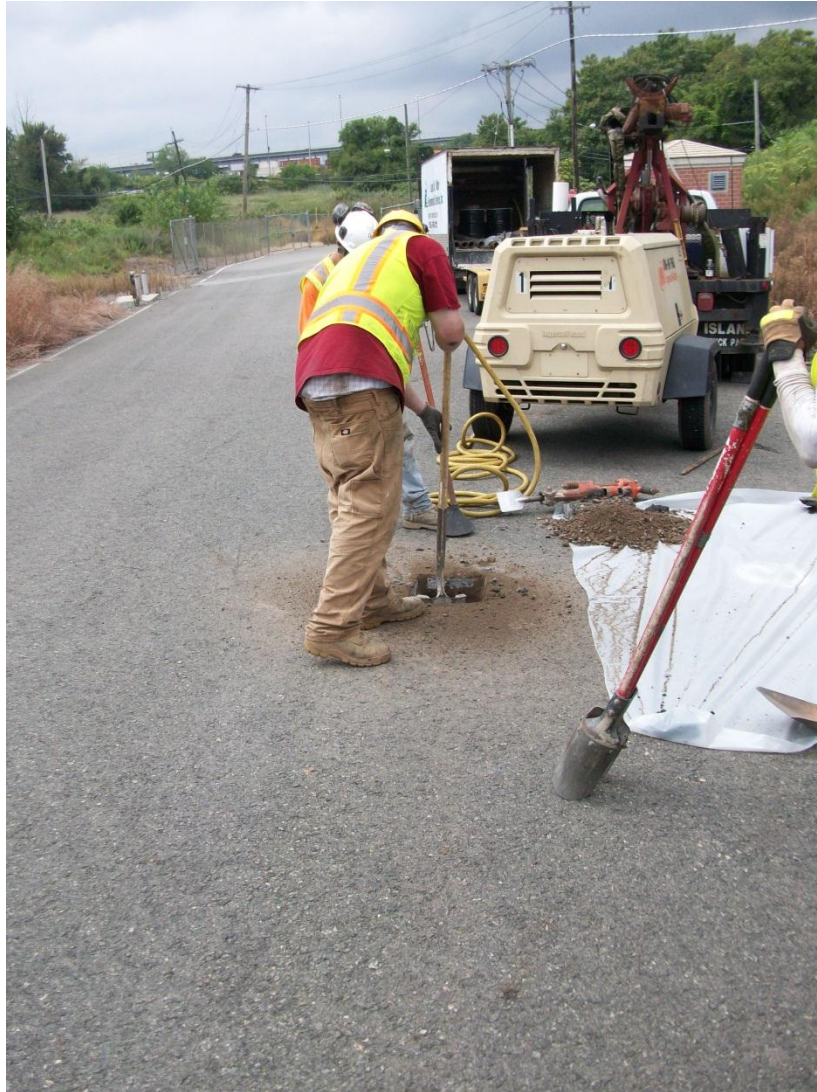
Figure 4: Hand-clearing the upper 6 ft of a boring
