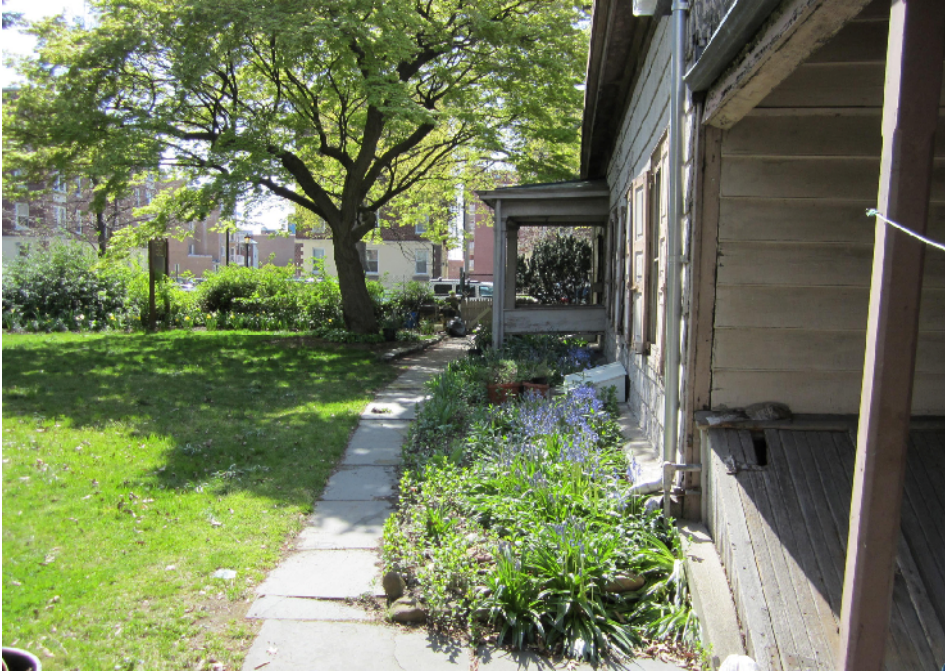
Photograph 11. View W from the walk along the S side of the kitchen wing. Note the concrete sill at foundation level between porch/cellar entrance and main entrance.
