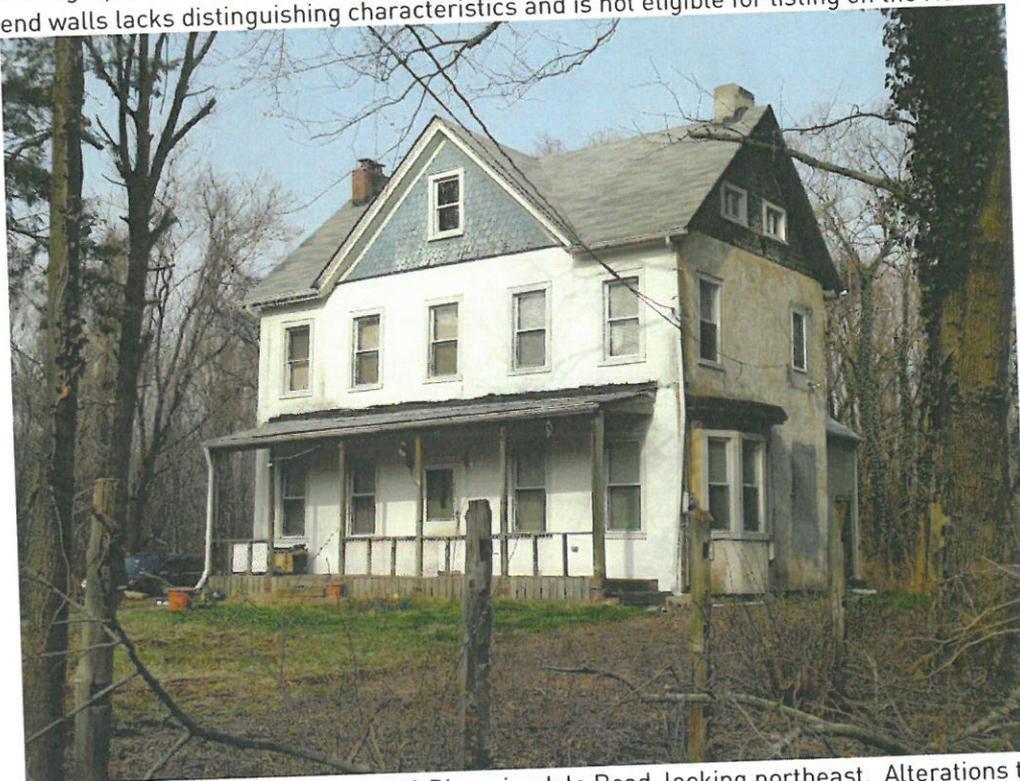
Photograph 38. Structure 104, 299 Bloomingdale Road, looking northeast. Alterations to the original fenestration pattern and porch have compromised the integrity of this dwelling; it is not eligible for listing on the National Register.
