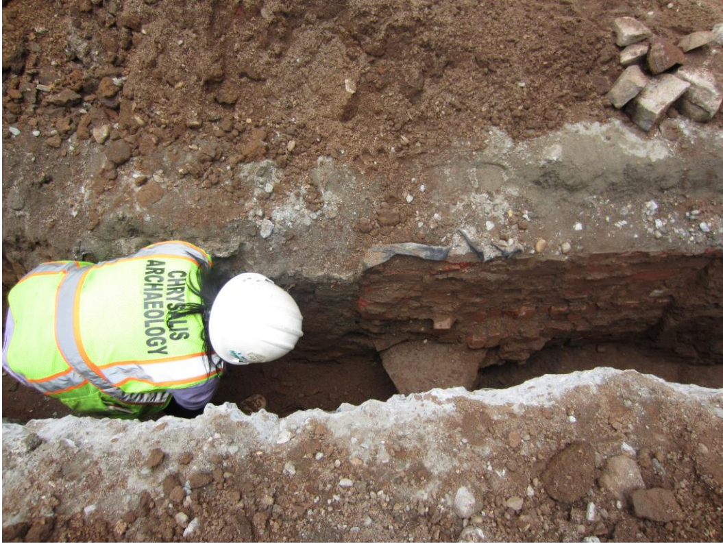
Image 09: Excavation the Water Line area
