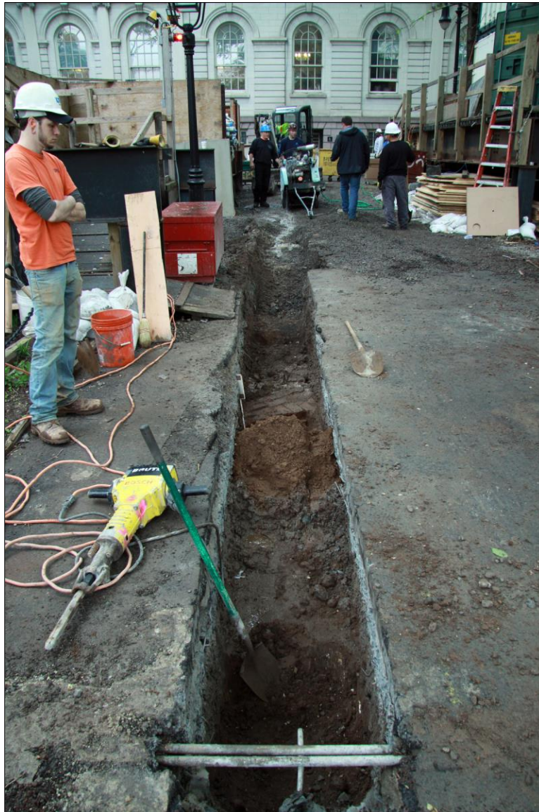
Image 03: Excavation along the Center Street/Park Row path, facing west.
