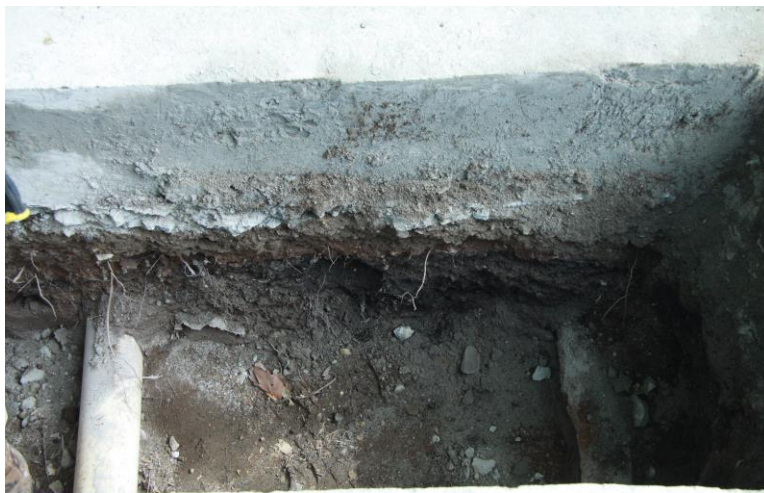
Image 02: Gas line work
