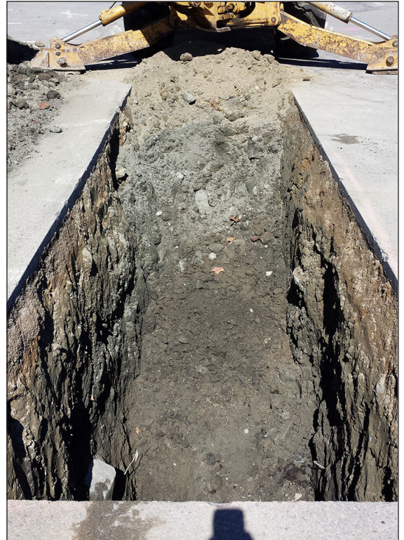
Facing northwest showing in progress excavation of Trench 2 5
