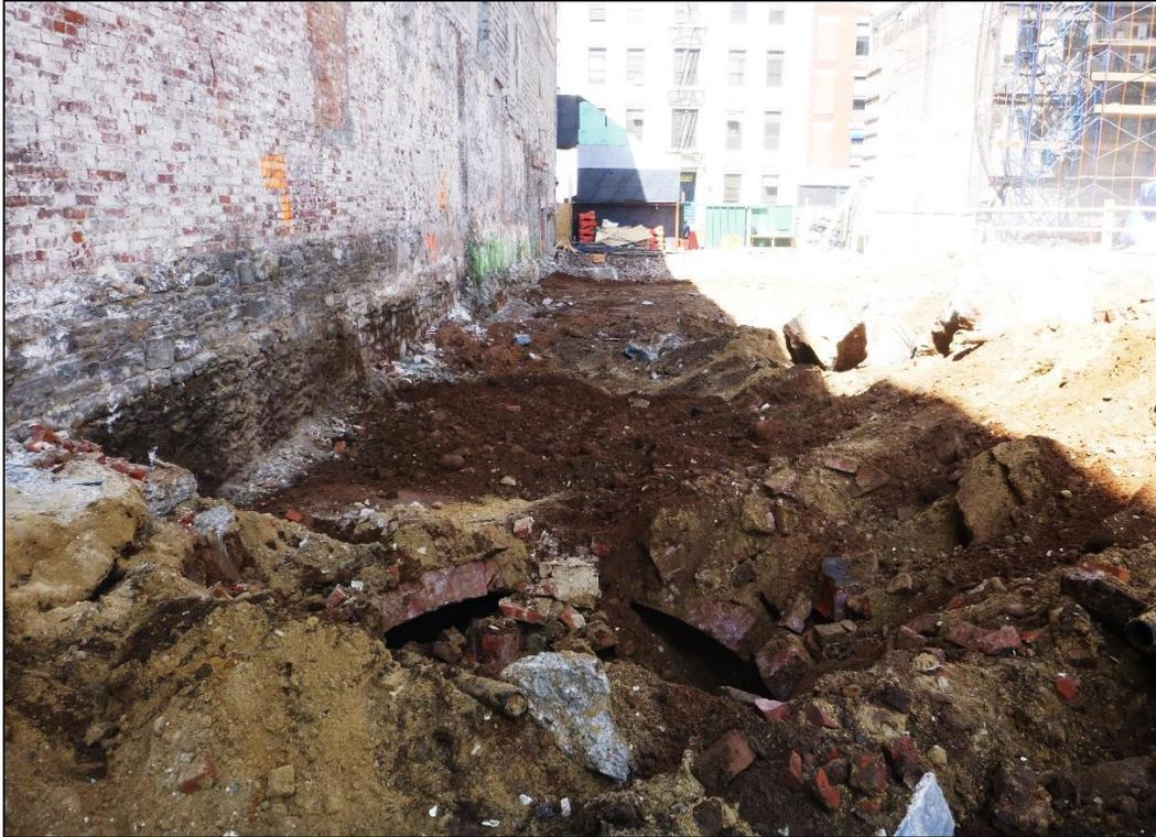
Image 09: Cistern with vaulted roof when first exposed.
