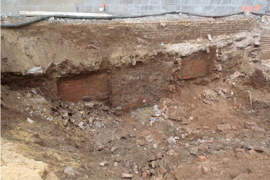
Image 01: Excavation of south wall of the Atlantic Garden basement showing both brick and stone wall segments.
