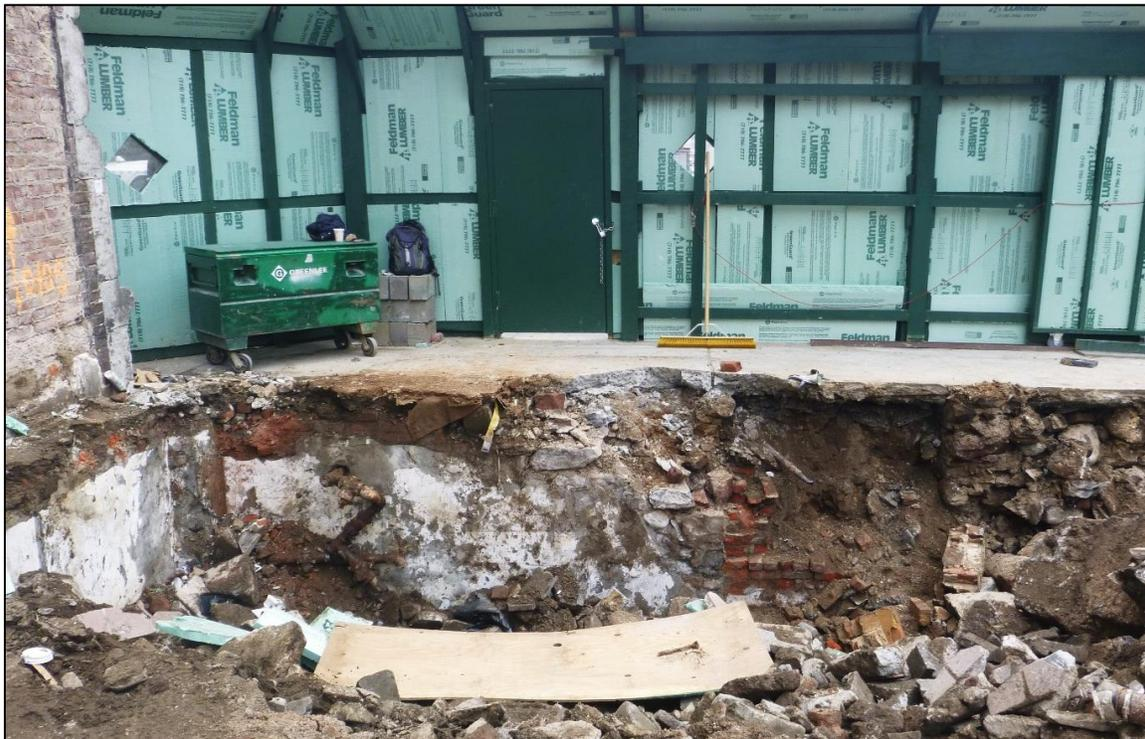
Image 16: Plastered fieldstone wall and brick wall from 52 and 52½ Bowery basements.
