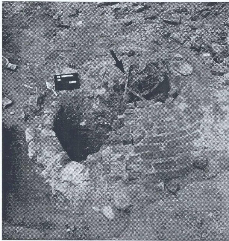
17 F8, a brick and stone beehive-domed water cistern at 78 MacDougal St. during excavation of its northwest quadrant. Note drain area (arrow), intact when tested in 1993, but broken during excavation for data recovery. (9/20/95)
