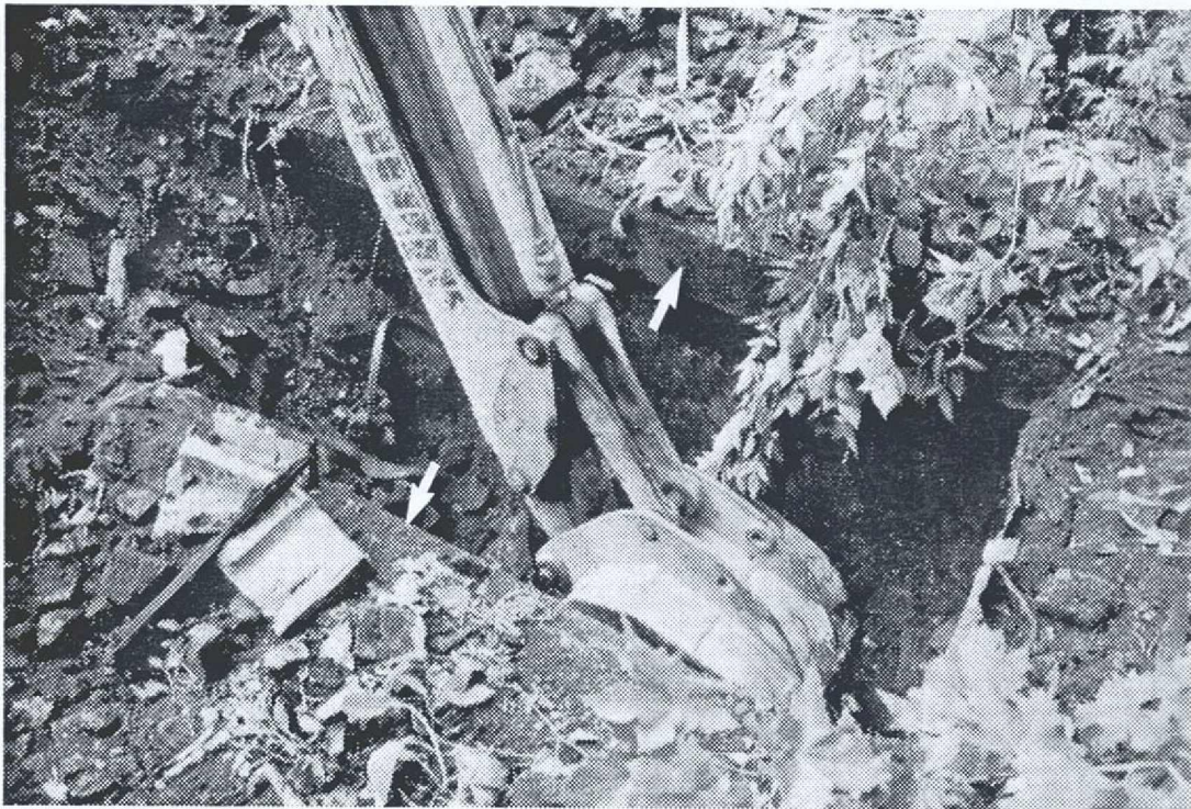
3 Backhoe excavation of test trench 1 (TT1). Excavation revealed a 4.3-ft. deep metal pit. Note metal "beams" (arrows) that proved to be part of the pit. (7/26/95)
