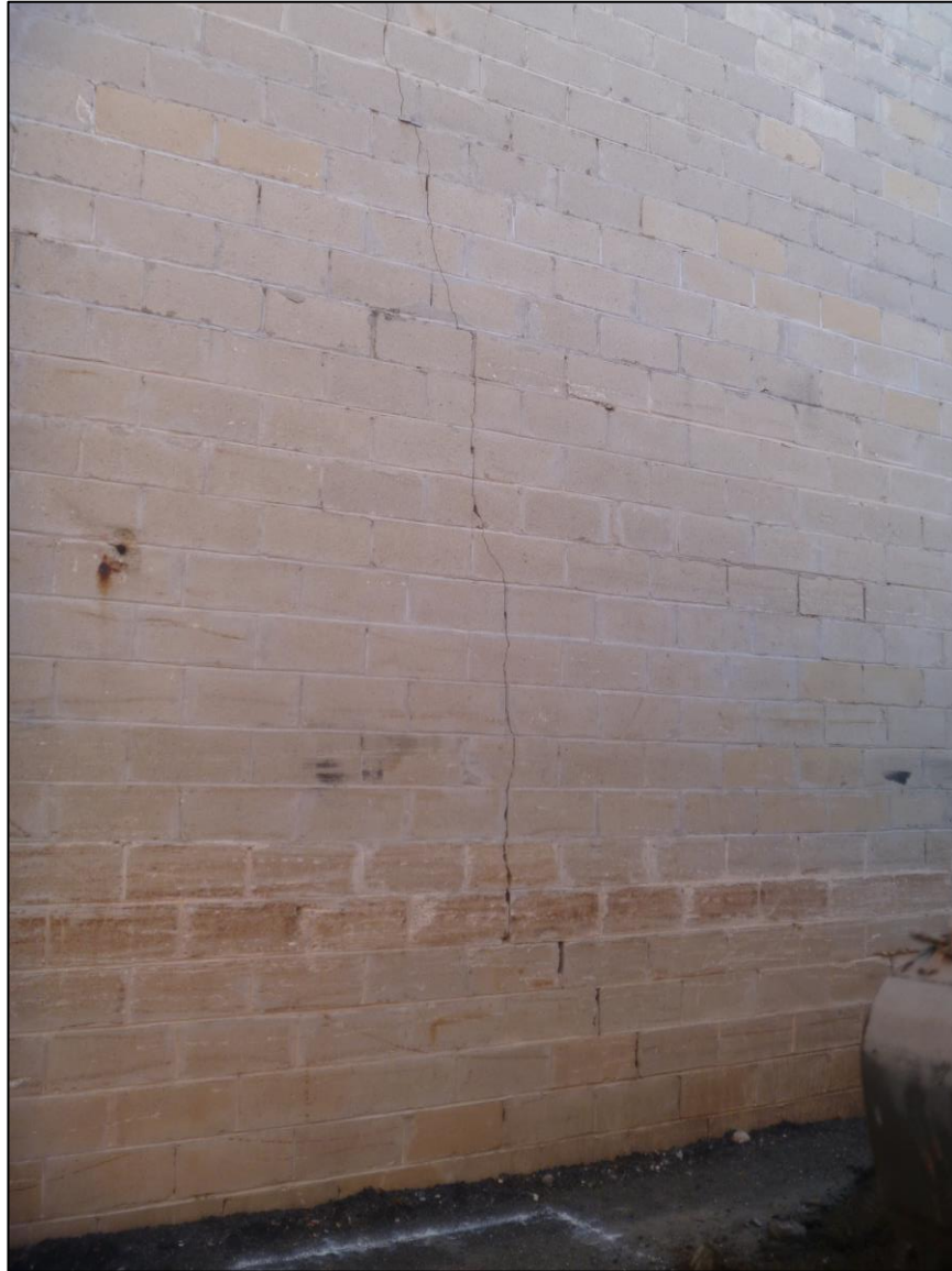
Image 03: Crack in the wall of the building neighboring the APE to the east.
