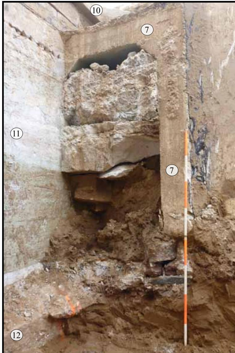
Photograph 3.21. Stair D Excavation Area: view looking southwest showing the cross-section of the tar-coated, concrete-encased, concrete-filled passage [7]; note the stone masonry at the base to the left of the scale rod; at left is the parade wall [11] set on a stepped battered mortared rubble base [12] and capped with coping stones [10]; scale in feet (Photographer: Joshua Butchko, March 2012) [HRI Neg.#11063/D13-50].
