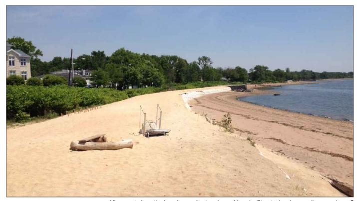
View east along the beach near the terminus of Loretto Street, showing sandbags and stone and concrete sea walls constructed along the waterfront.
