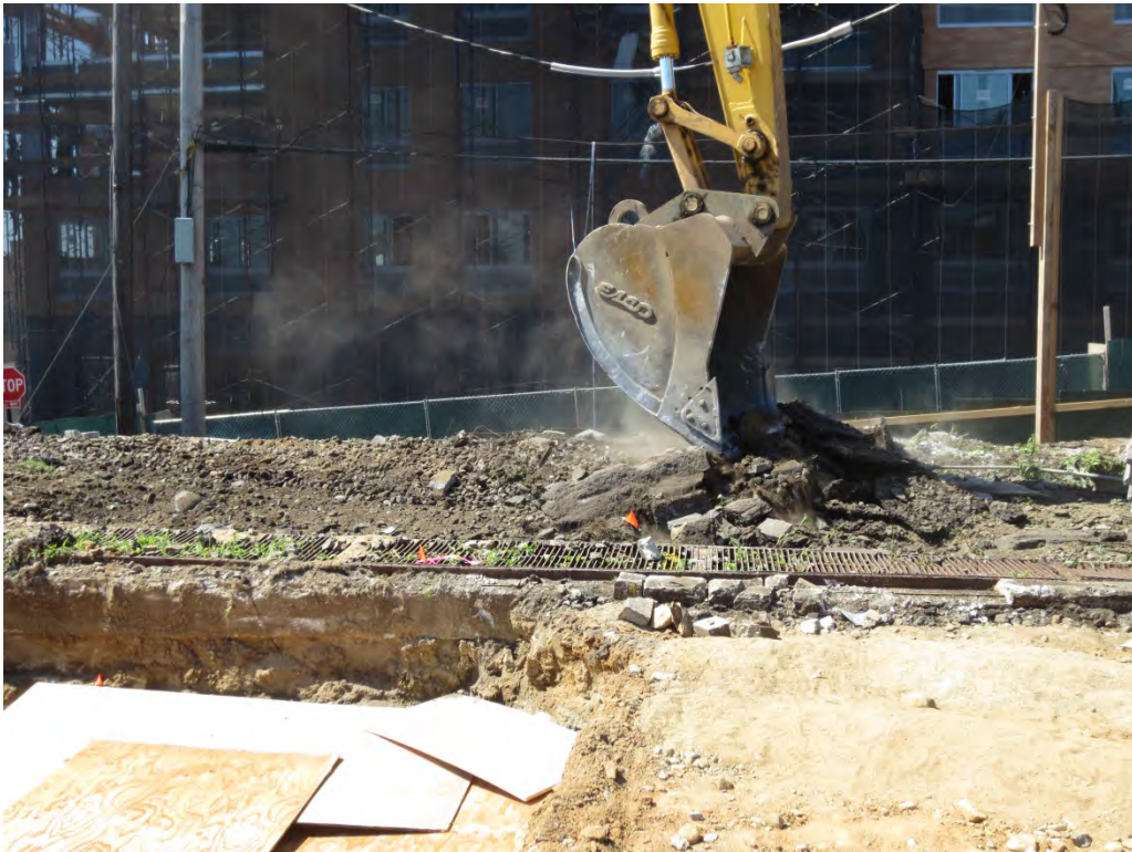
Photograph 1.5: South end of Block 3014 showing French drain parallel to East 172 nd Street, view to south during site excavations.
