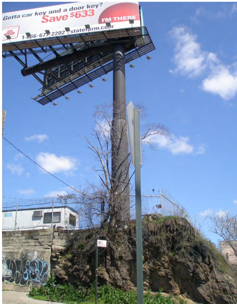
Photograph 1.3: Billboard at southeast corner of Block 3014, with post and footings on bedrock, view to north.
