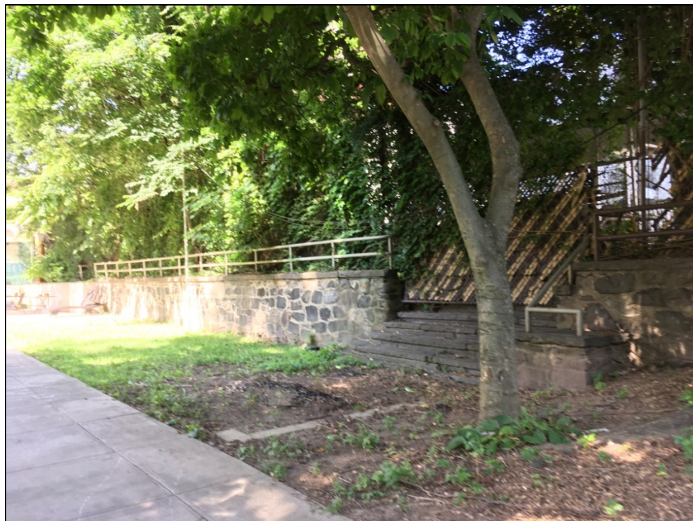
Photo 12: View northeast from Lot 19 towards rear of Lot 37, showing north-south oriented stone party wall between the lots; note the bluestone stairway, at right, along the south end of wall.
