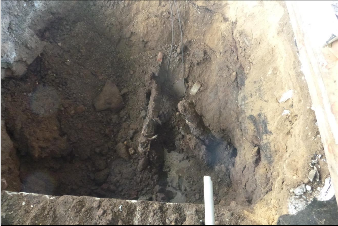
Image 08: Possible cribbing timbers in Trench CB-11.
