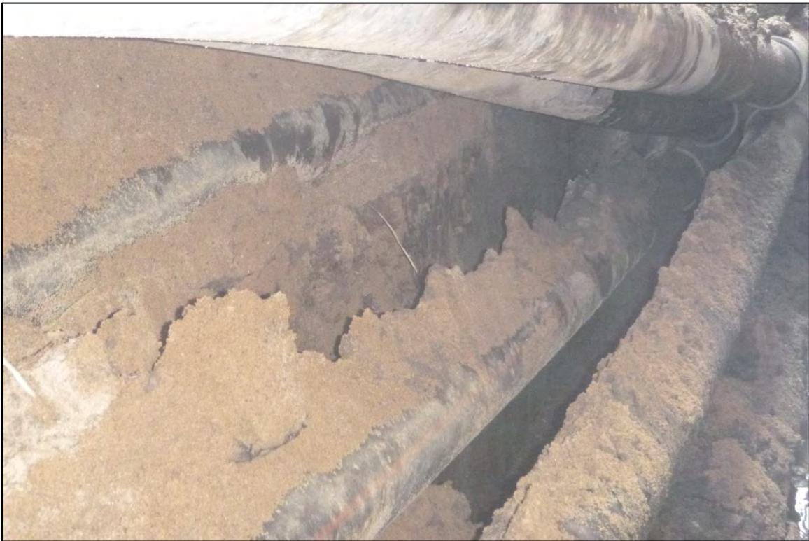
Image C.27: Trench 6 – Feature 3, zoom view of bulkhead beneath ConEd feeders in west wall.
