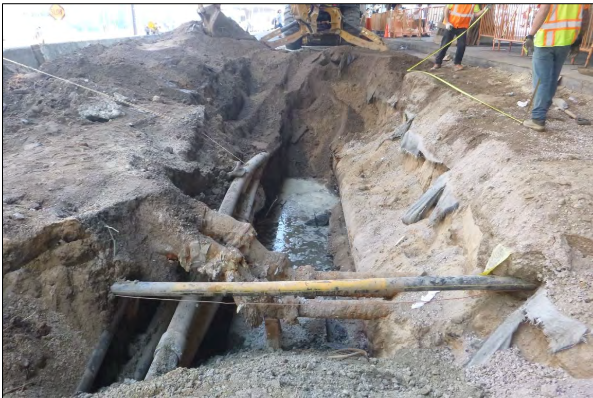
Image C.33: Trench 7 – plan view in progress, heavy utility disturbance.
