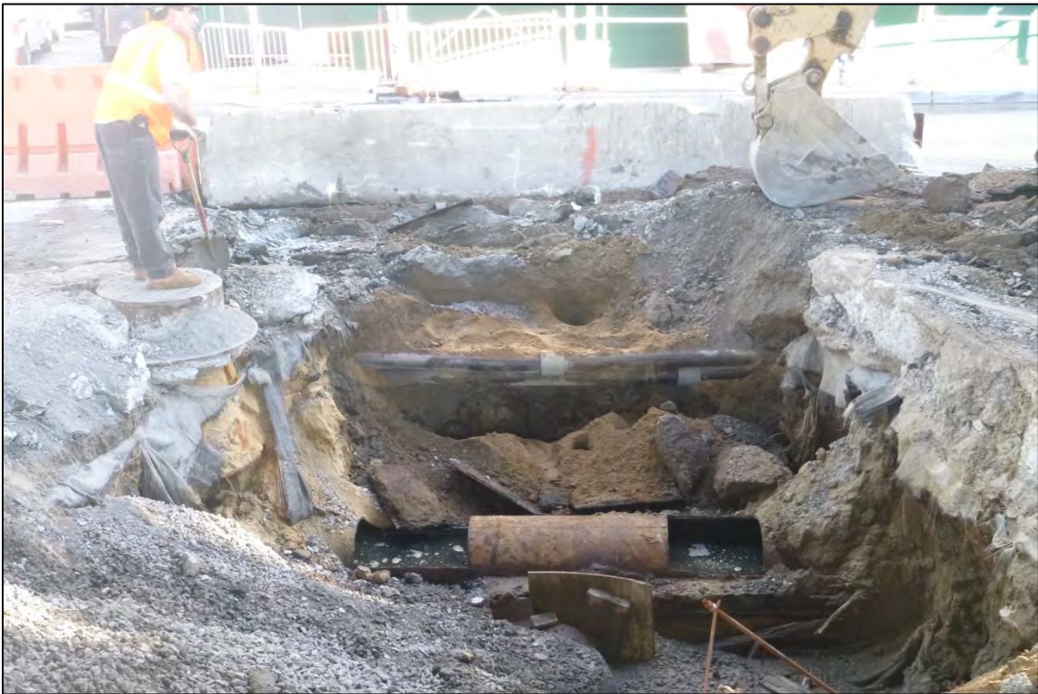
Image C.17: Trench 4 – west half, ConEd feeders in west profile.
