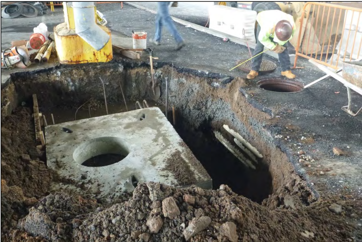
Image C.05: Trench CB-7 – catch basin installation.
