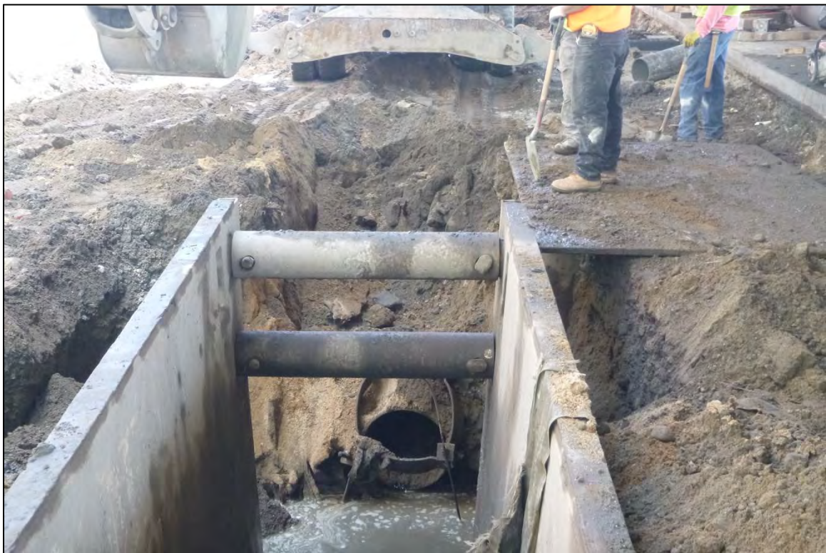
Image C.23: Trench 6 – excavation in progress, old WM in base of trench, facing north.
