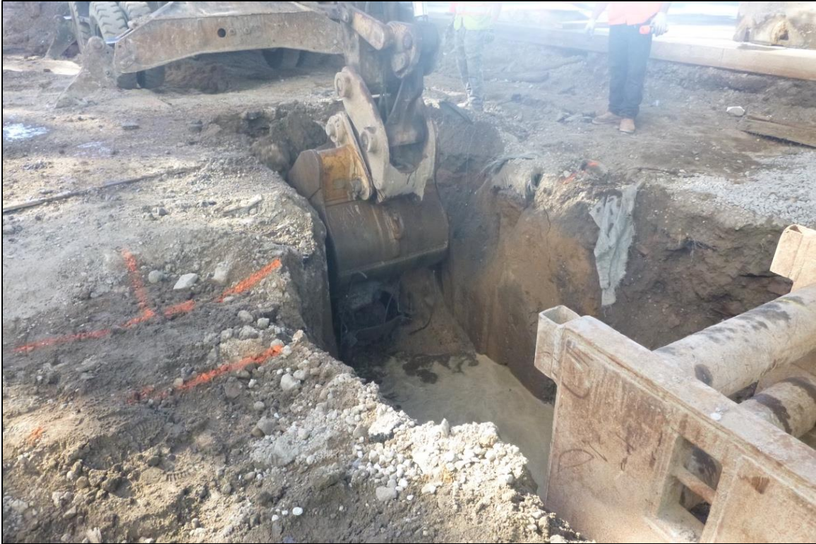
Image 18: Trench 5 shifted a few feet eastward towards the curb to mitigate intrusion by the large concrete manhole between 38.5' and 54' north of Column #19.
