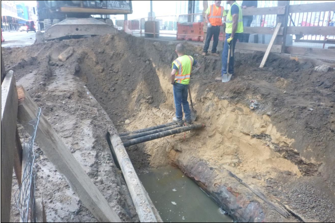
Image 28: Trench 8, excavation in progress. Stratum II surrounding 20" WM in East Profile.
