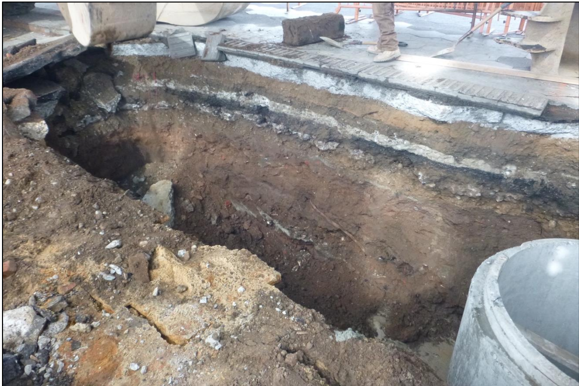
Image 11: Trench 2 East profile from MH #10 to 27' N, brick and mortar at 6' bgs.
