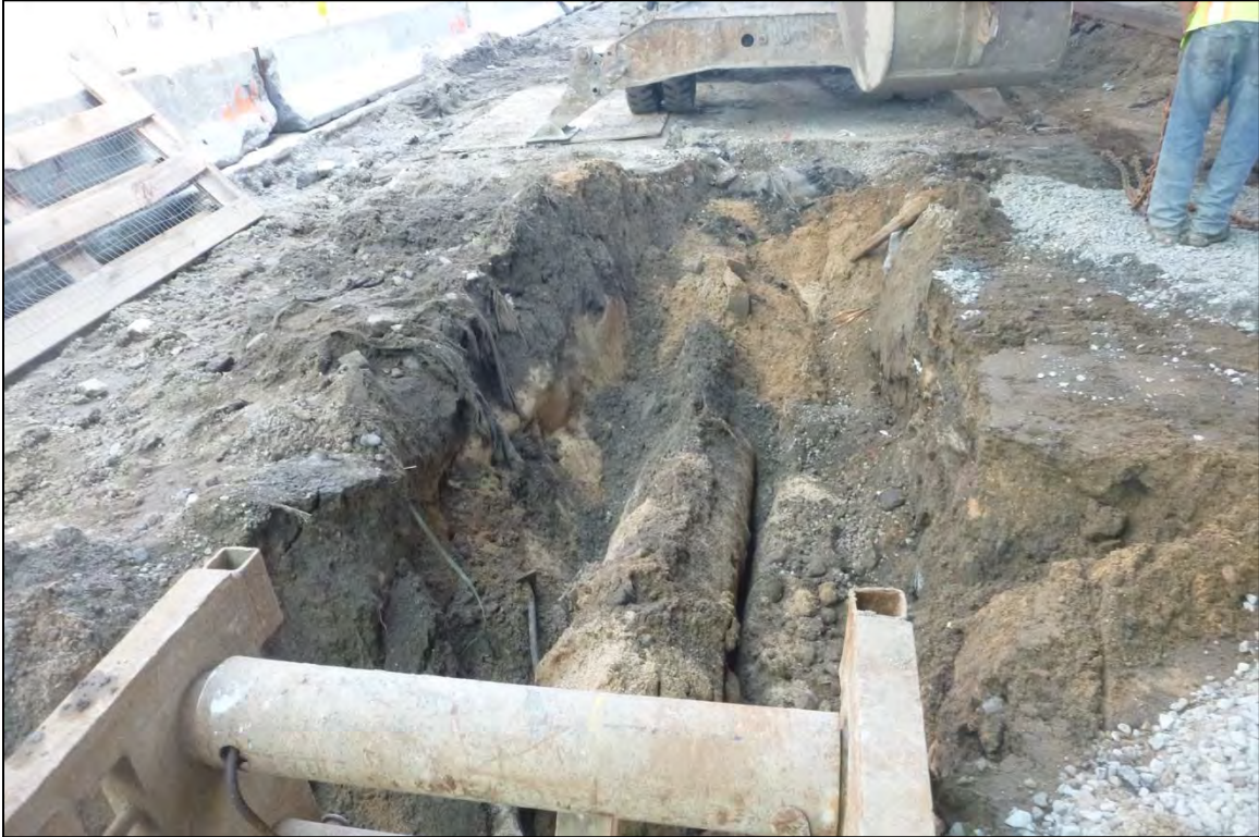
Image C.18: Trench 5 – excavation in progress, old WM in center of trench, facing north.
