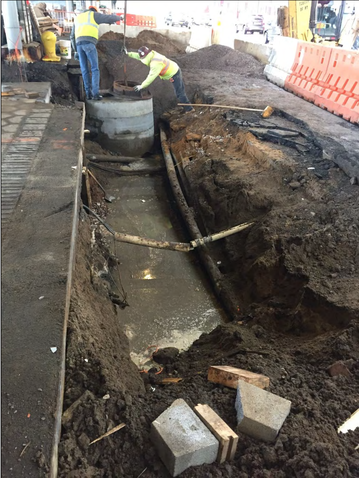
Image C.03: Trench 1 – Plan view in progress, ConEd feeders in west profile
