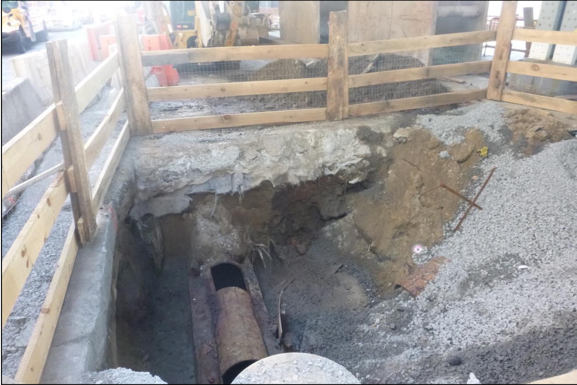
Image 15: Trench 4 excavation upon arrival on site, eastern portion backfilled behind new pipe.
