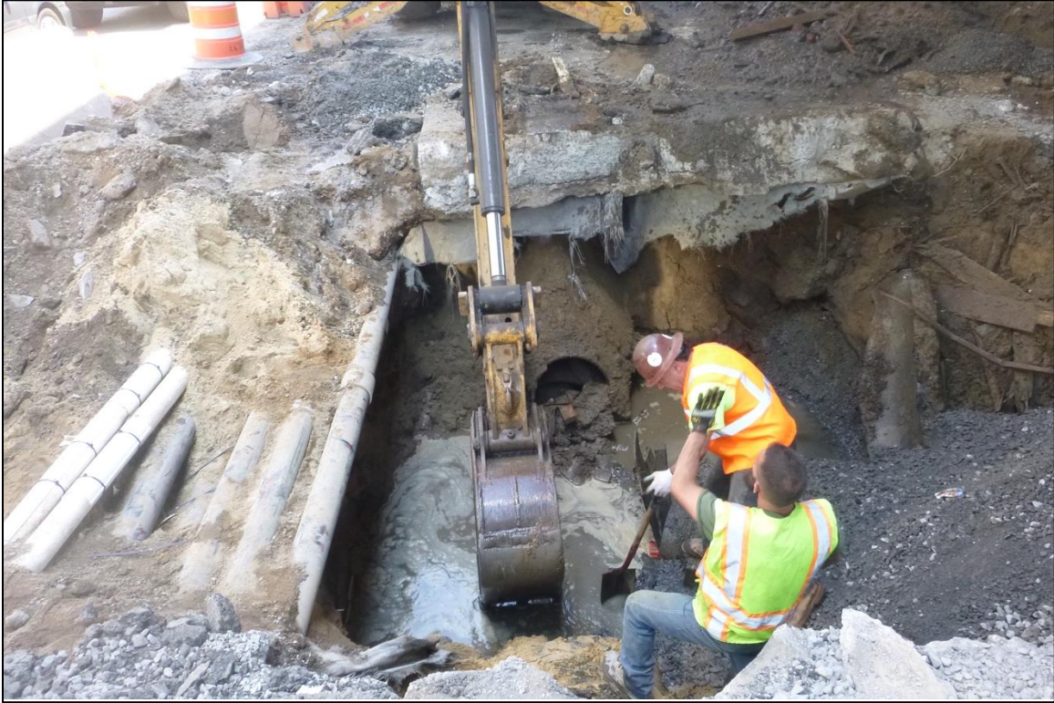
Image 17: Excavation in the space between 20" water main and western expansion, which exposed ConEd feeders, from 15.5' west of east curb line to 18.5' west of east curb line.
