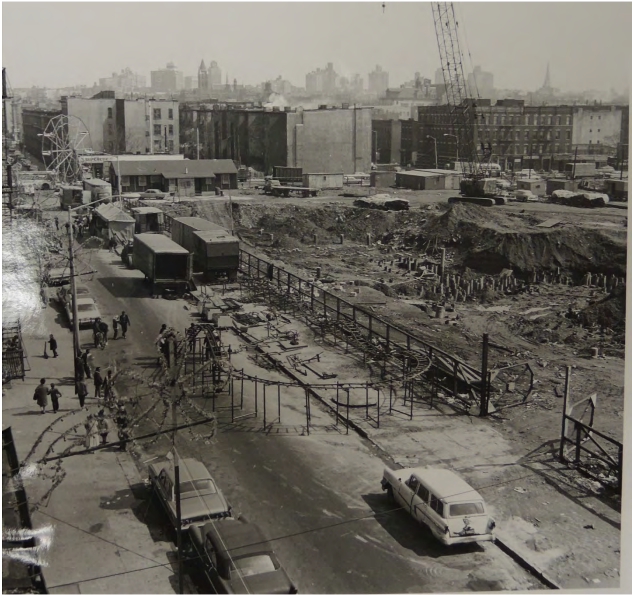
Historic Photograph 4: NYCHA excavations for Wyckoff Gardens, facing east to excavations for Building 3. Wyckoff Street (with amusement rides) is in foreground and Third Avenue is in background. Note that excavations extend north to Wyckoff Street and south to mid-block, encompassing most of the eastern Area of Potential Effect, although there appears to be a small, undisturbed area immediately adjacent to Third Avenue where a building office and several vehicles are sited (NYCHA Photo 02.015.11620, 4/9/1965).
