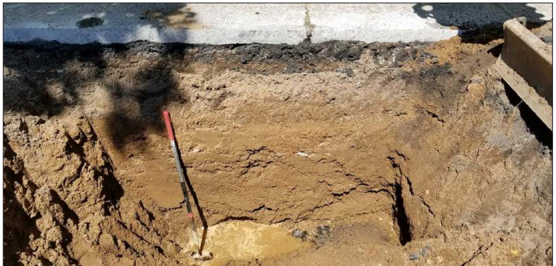
Facing southwest showing west wall of the southern half of TP3. Note clean fill with no evidence of wall remains and water accumulation on trench floor at about 6 feet bgs
