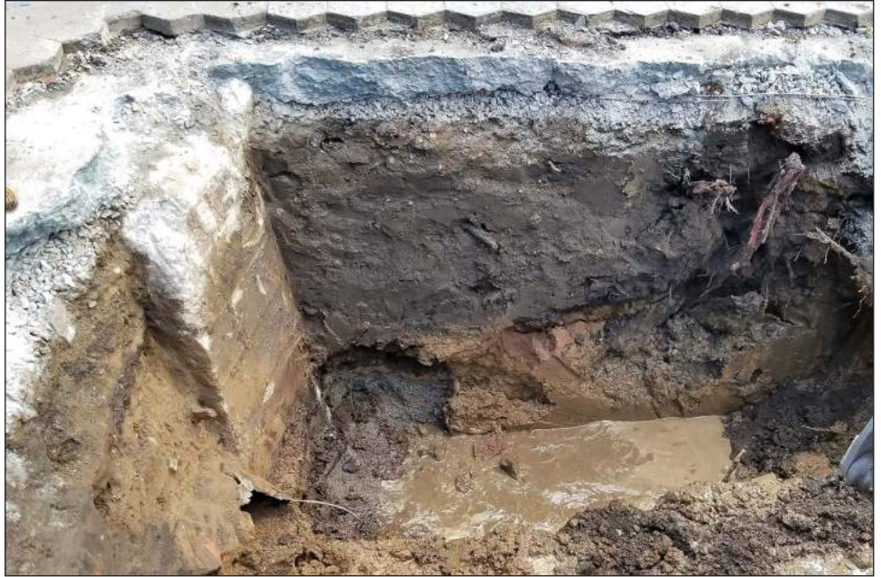
Facing north at the west end of TP1 showing the north wall profile and poured concrete pier to the left. Note that the floor of the trench is filling with water at a depth of about 6 feet bgs
