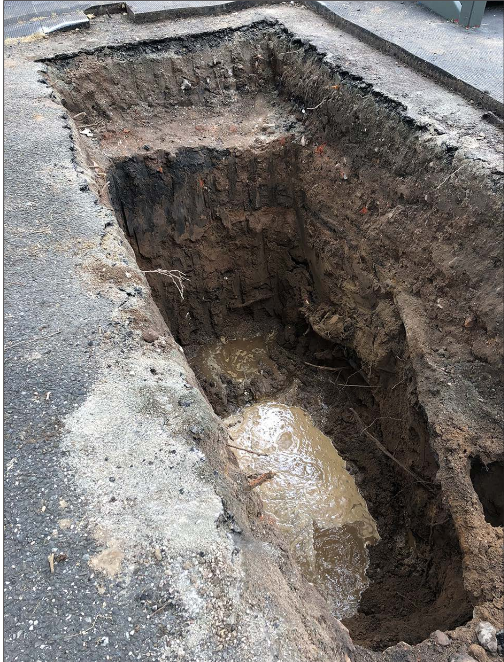
Facing south showing southern half of TP9. Note utility line extending through trench along the right side of photo and the accumulation of water on the trench floor at a depth of 6 feet bgs. Not visible in this photo are two dressed stones encountered just below the water surface which appear to be part of an intact foundation wall
