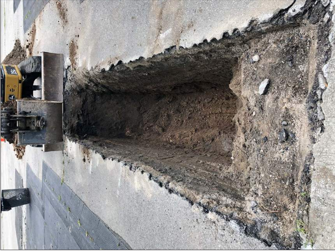
Facing south showing excavated TP7, which consisted of clean sandy fills 23
