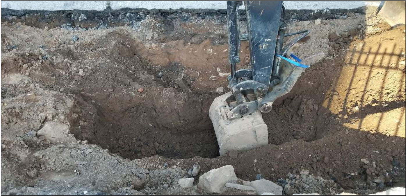
Facing southwest showing deeper excavation of northern half of TP3. No additional stones were encountered to a depth of 6 feet bgs
