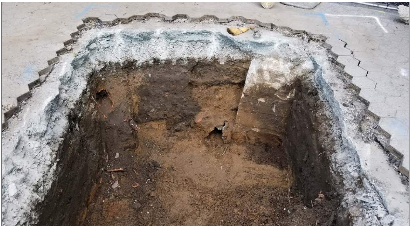
Facing west towards western wall of TP1. Note 6-foot-tall poured concrete pier in northwest corner of trench, disturbed soils, and fractured drainage line in southwest corner of trench. The trench floor is approximately 4 feet bgs in this photo
