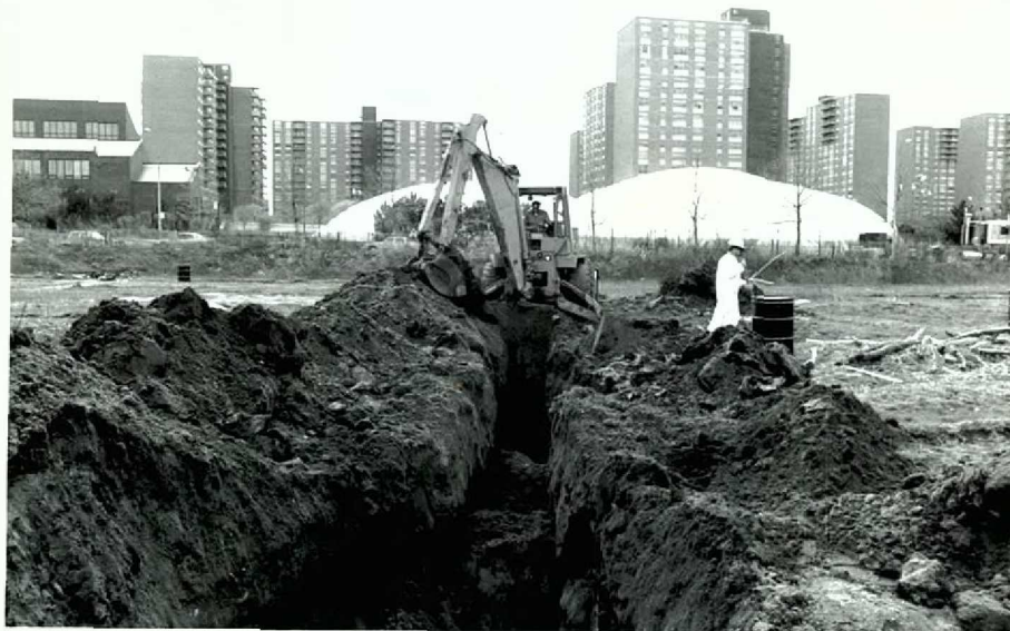
PLATE 1: View of backhoe trenching in operation.
