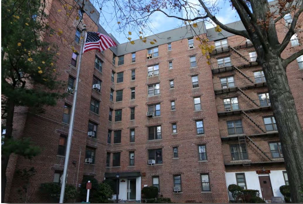
Plate 7: Detail view of the Dorie Miller Cooperative Houses (RGA112) showing replacement windows and reconstructed brick lintels.
