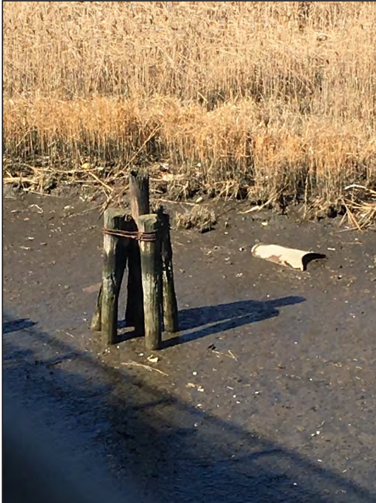
Photo 5.7: Wooden mooring structure (dolphin) in the tidal wetlands adjacent to Flushing Creek adjacent to the MTA/Tully Site Stormwater Outfall APE- Archaeology at Flushing Creek, observed from the Roosevelt Avenue Bridge.
