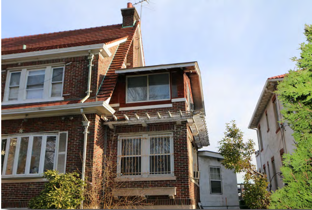
Plate 3: Detail view of number 105-05 (RGA100) showing the one-story brick wing with trellis, modern enclosure on the sleeping porch, and the one-story concrete block addition.
