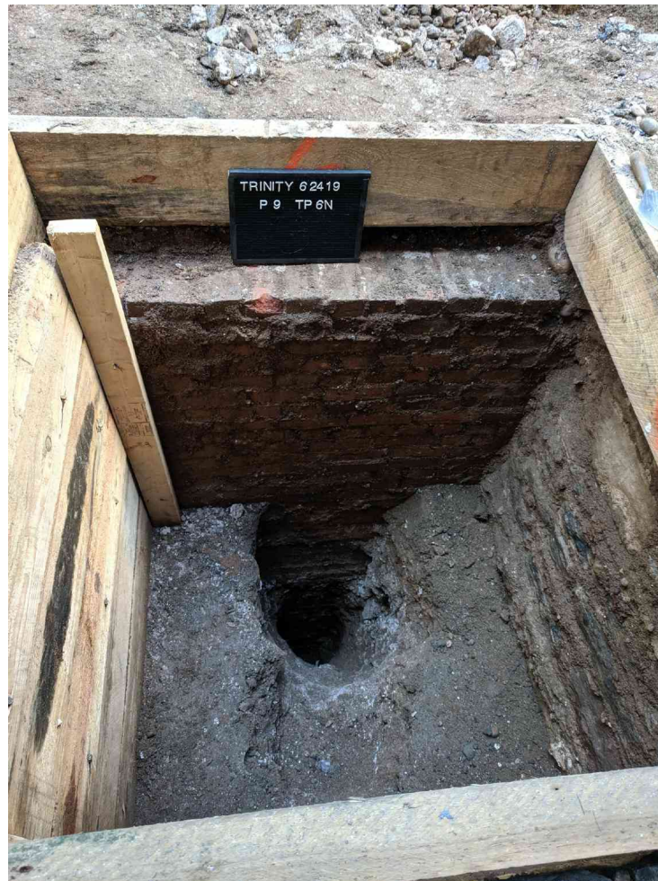
Photo 37. TP 6N and the site for Pile 9 excavated to 9.8 ft. (3.0 m) BGS. The view is south. The pile site is adjacent to the brick vault wall first noted in TP1. Fill included whiteware frags and a corroded nail. Construction to the right, which defines the west TP wall, was unidentified. (D. George 6/24/19)
