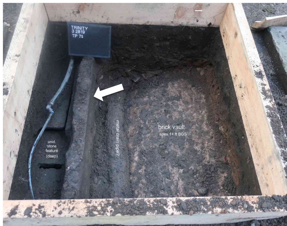
Photo 40. Annotated view of TP 7S after excavation exposed a burial vault, a cast-iron drain pipe, what proved to be the stone edging (arrow) of vault access, and overlapping stone slabs (the view is south). (J. Geismar 3/28/19). The slabs were fully uncovered (see Figure 19) and, with the church's consent, the site for Pile 8 was relocated to the access to avoid disturbance to the burial vault.
