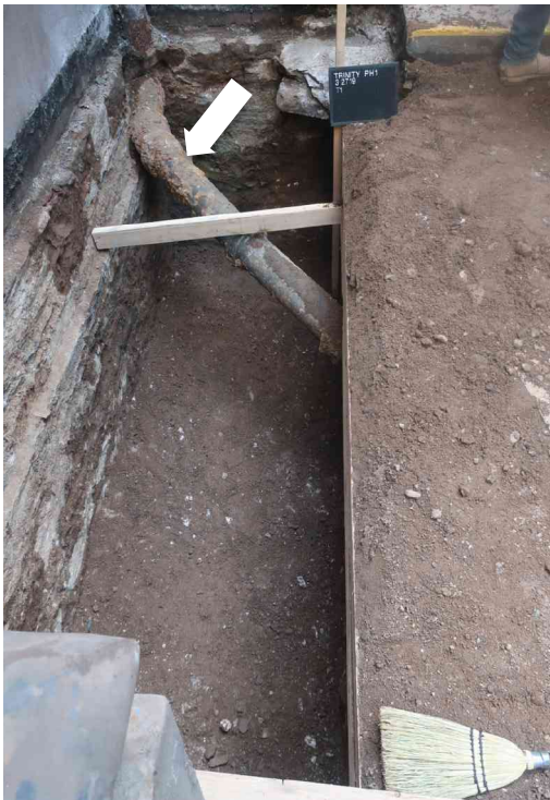
Photo 24. TP 1 in the easternmost alcove. A Cast-iron drain pipe (arrow) is exposed in the east end of the TP. (J. Geismar 3/27/19)
