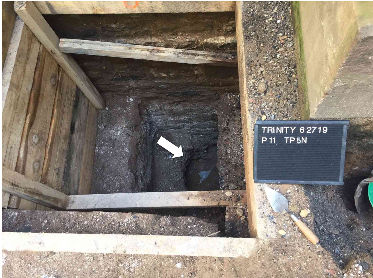
Photo 34. TP 5N after excavation to test for Pile 11. While there was no archaeological oversight beyond 6 ft. (1.8 m) BGS, the photo, taken 6/27/19, suggests the test was at least 9 ft. (c 2.7 m) BGS. (J. Geismar 6/27/19)
