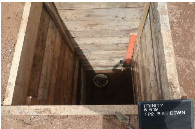
Photo 28. TP 2 after extension from its original 4 ft. (1.3 m) depth to 10 ft. (3.1 m) BGS with archaeological oversight (J. Geismar 6/6/19). An additional 15 ft. (4.6 m) were added without oversight to fulfill a Building Department requirement. Lagging covers the vault wall exposed on the east side (right) of the TP. Note the bucket (arrow) in the northwest corner of the TP.
