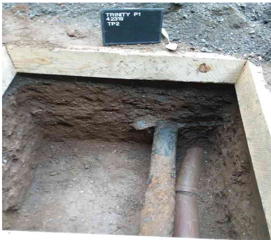
Photo 27. TP 2 with cast-iron (left) and terra-cotta (right) pipes exposed on the west side of the TP. The view is south. (S. Spritzer 4/23/19)
