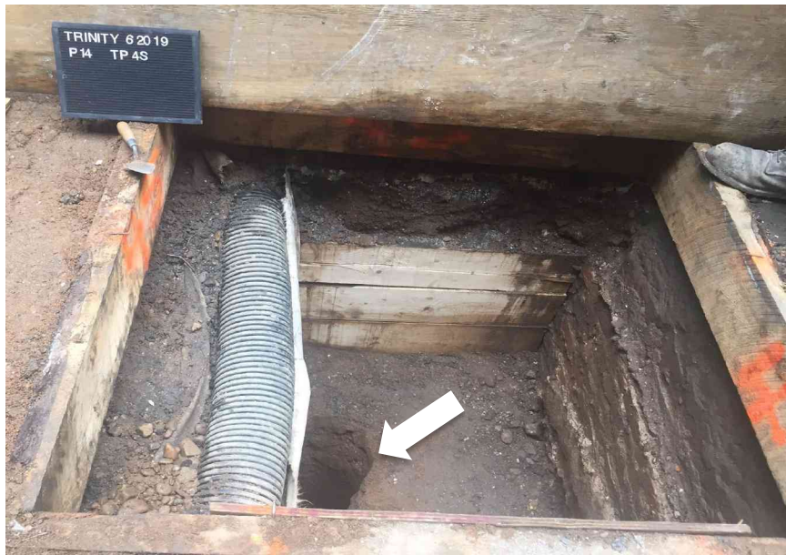
Photo 33. TP 4S after pile site excavation with a post hole digger. The PVC pipe on the east side of the TP was exposed during the earlier TP excavation and was left in place. What appears to be a vault wall is to the right. The view is south. (J. Geismar 6/20/19)
