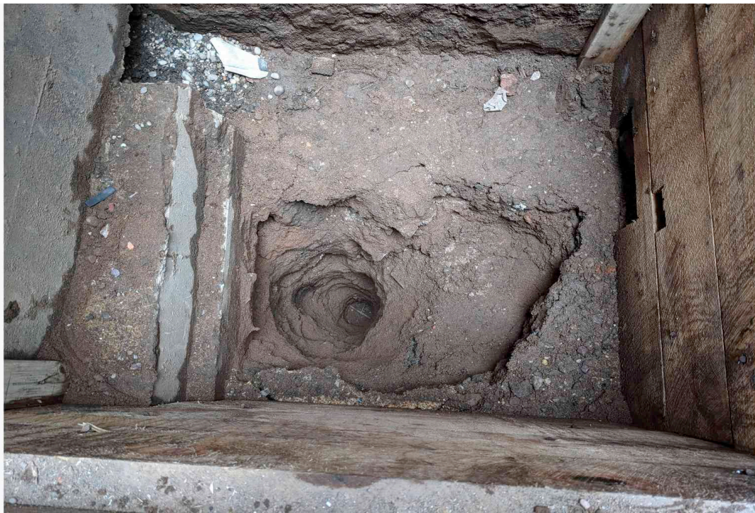
Photo 48. Completed excavation to 9.8 ft. (3.0 m) BGS of test for Pile Site 1 in TP 10 is a good visual example of a pile test excavation. (D. George 6/24/19)
