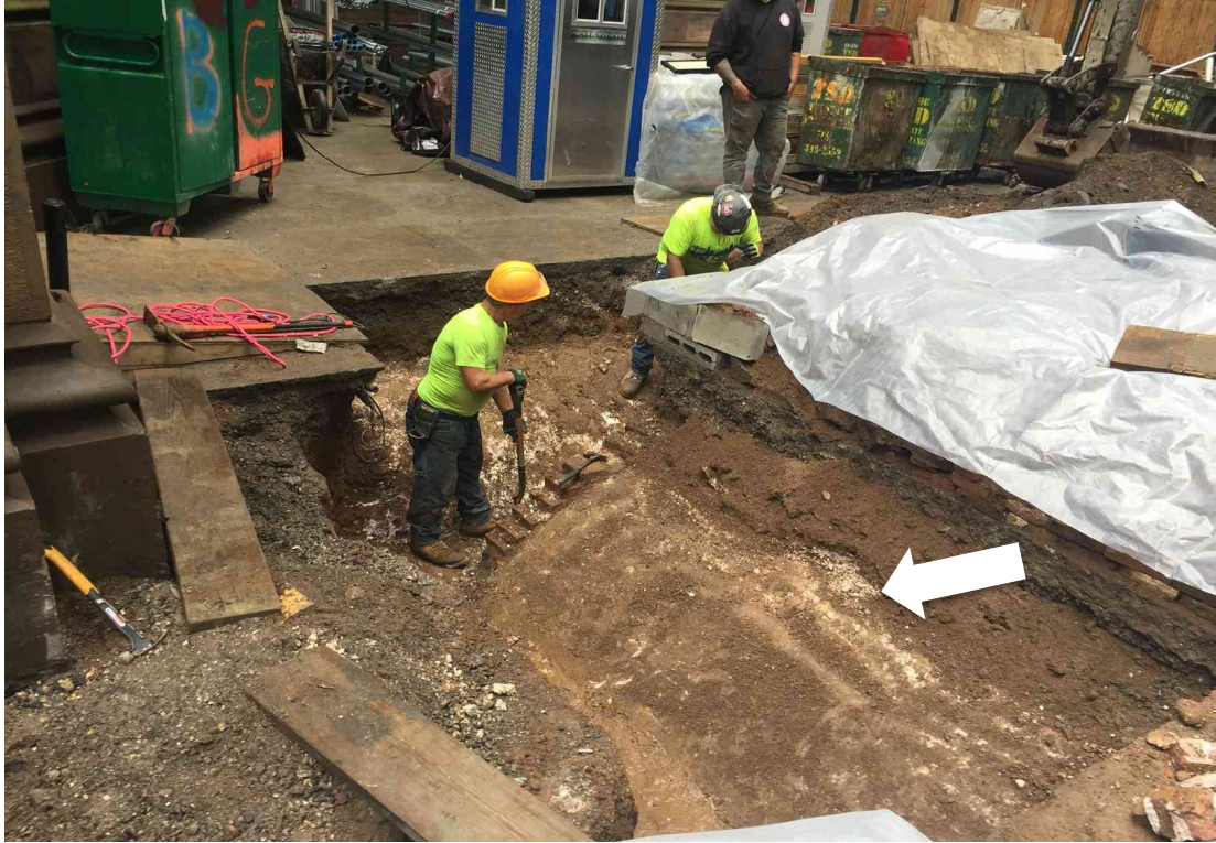
Photo 54. Drainage trench excavation in the vicinity of Wynant Van Zandt's large brick burial vault (arrow). Soil and cinder block were introduced above the vault. (J. Geismar 8/28/19).
