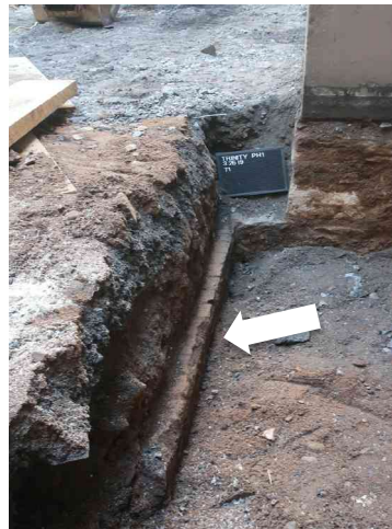
Photo 25. Top of brick vault "wall" (arrow) exposed on the south side of the TP. (J. Geismar 3/26/19)
