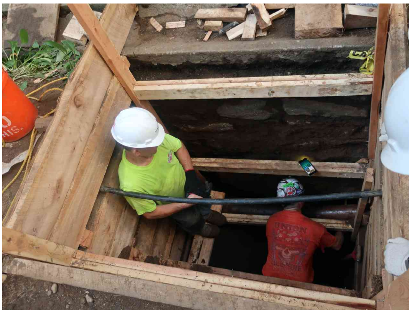
Photo 21. TP 9A, located adjacent to the Rector Street exterior wall and east of TP TP 9 and TP 9 EXT, near the end of excavation by LIC personnel. Lagging was introduced sequentially to shore the test Pit that ultimately extended down 11.9 ft. (3.6 m) BGS to expose the exterior wall footing and a pier-like inner wall. Scattered human remains were recovered from fill between 2.0 to 4.0 ft (0.6 to 1.2 m) BGS. (J. Geismar 8/31/18)
