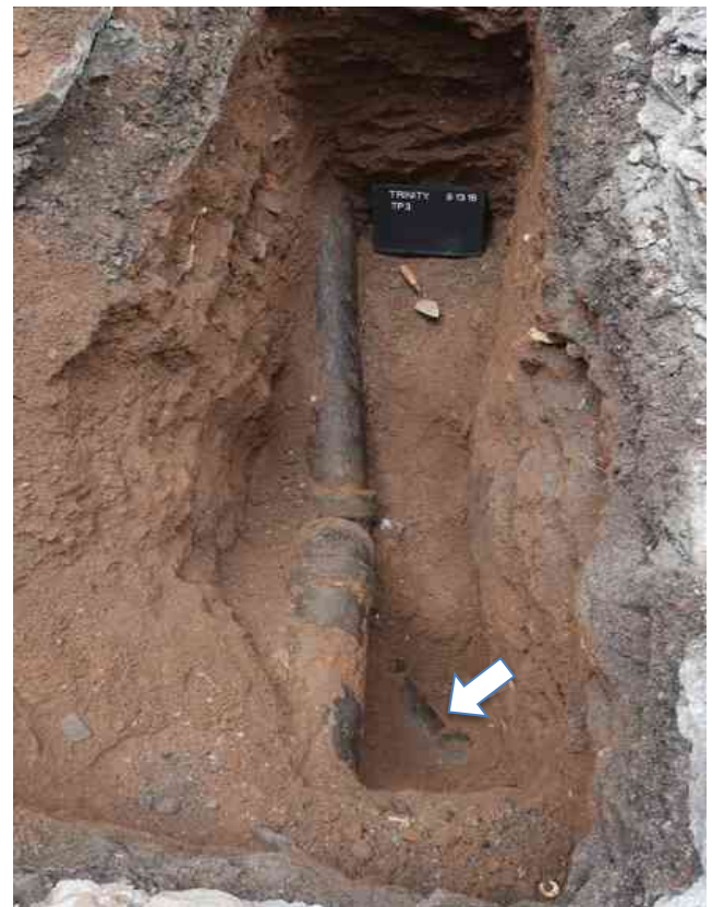
Photo 12. A network of relatively recent drain pipes, the sought after utilities, exposed in TP 3 on the south side of the church. Note a partially exposed deep pipe segment (arrow) to the right (J. Geismar 9/13/18)
