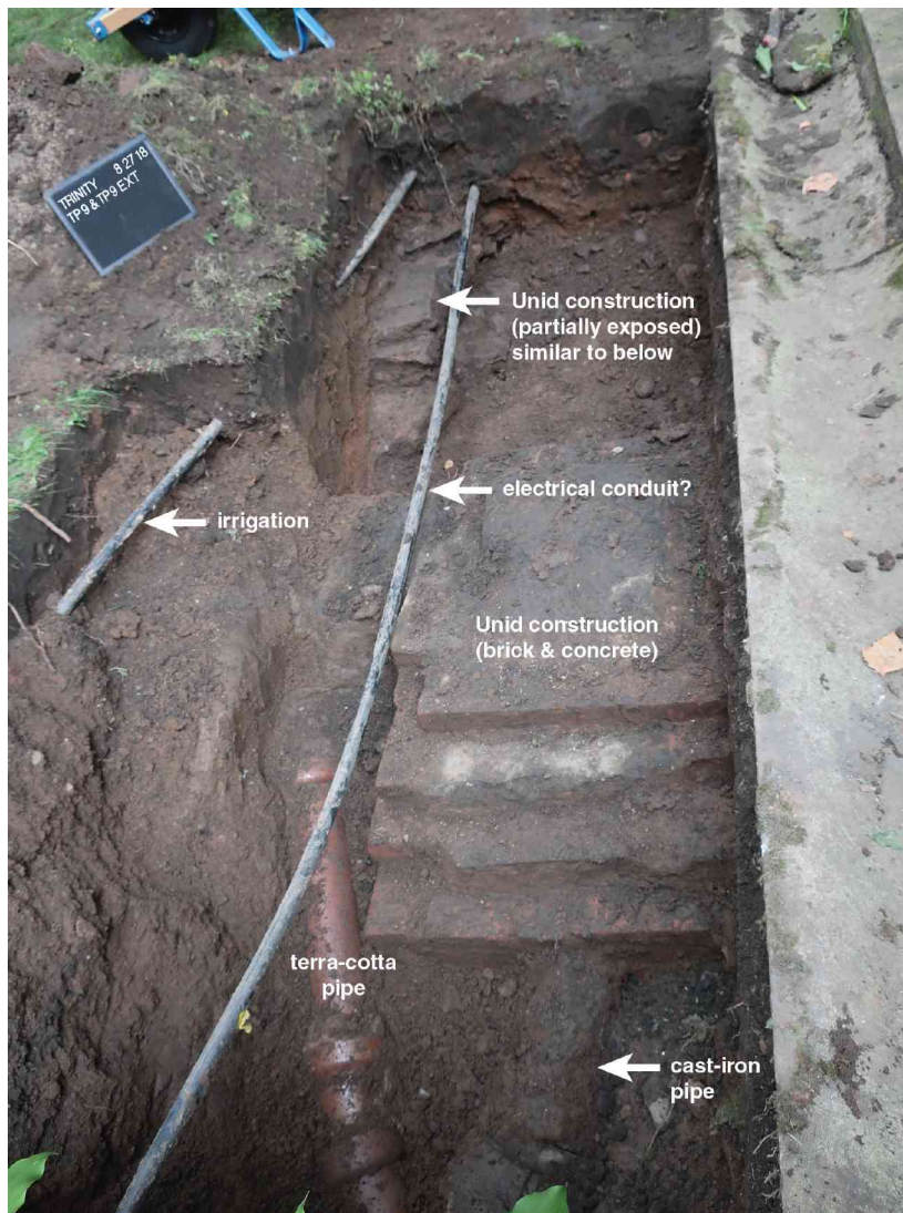
Photo 20. TP 9 and TP 9 EXT looking east. Two similar drainage features are exposed: the step-like brick construction to the right (adjacent to the Rector Street wall) with an associated cast-iron pipe and a terra-cotta pipe (left foreground) associated with a similar brick construction (only partially exposed) in the upper left corner of the pit. An irrigation pipe (far left) and a probable electrical conduit (center) complete the picture. (J. Geismar 8/27/18)
