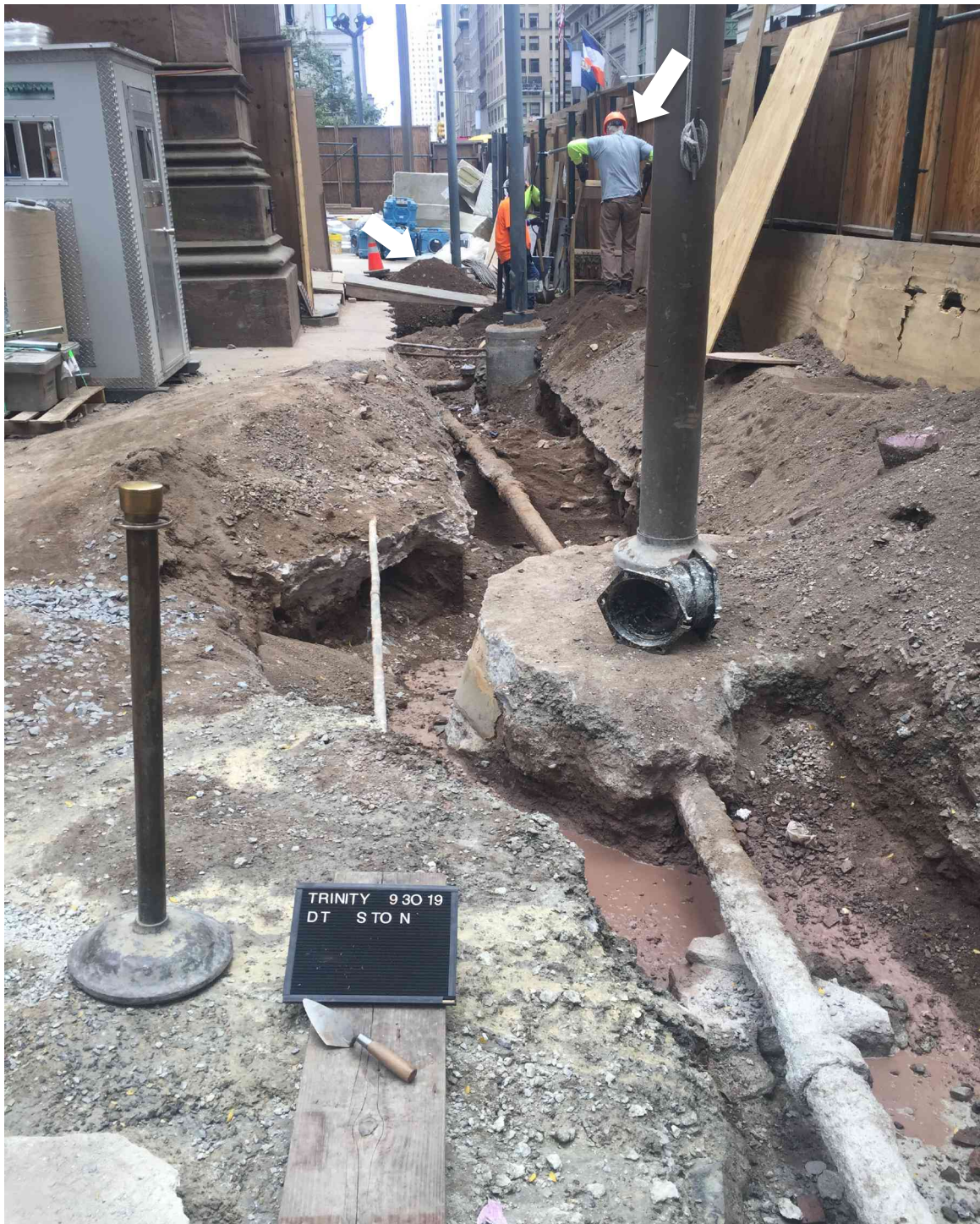
Photo 56. The north-south leg of the drainage trench looking north. A cast-iron pipe is exposed in the trench and Broadway is to the right beyond the plywood and chain-link fence. The excavated soil is being screened in the very limited space between the trench and the fence (right arrow). Excavation terminated to the north, just beyond the church's Broadway entrance where some screened soil temporarily is stockpiled (left arrow). (J. Geismar 9/30/19)
