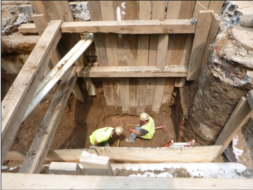
Image 31: Trench 2 Section 11 – Sewer at 8.28' NAVD88 (12' bgs).
