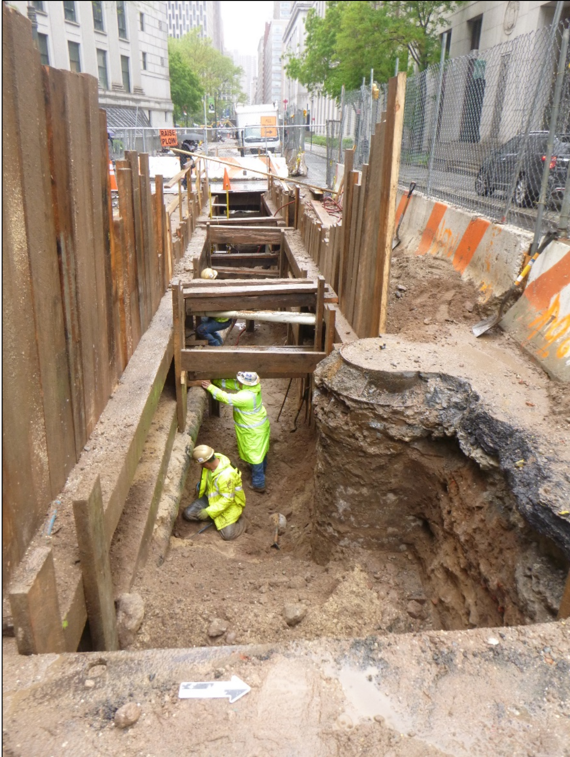
Image 30: Trench 2 Section 11 – Brick manhole in north wall.
