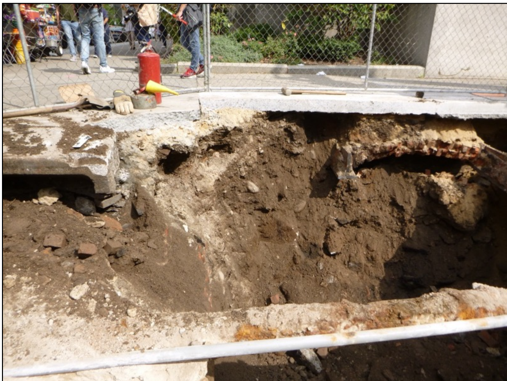
Image 58: Trench 16 Section 1 – Vault below sidewalk.
