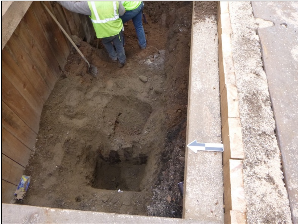
Image 18: Trench 2 Section 4 – Old sheeting in test pit.
