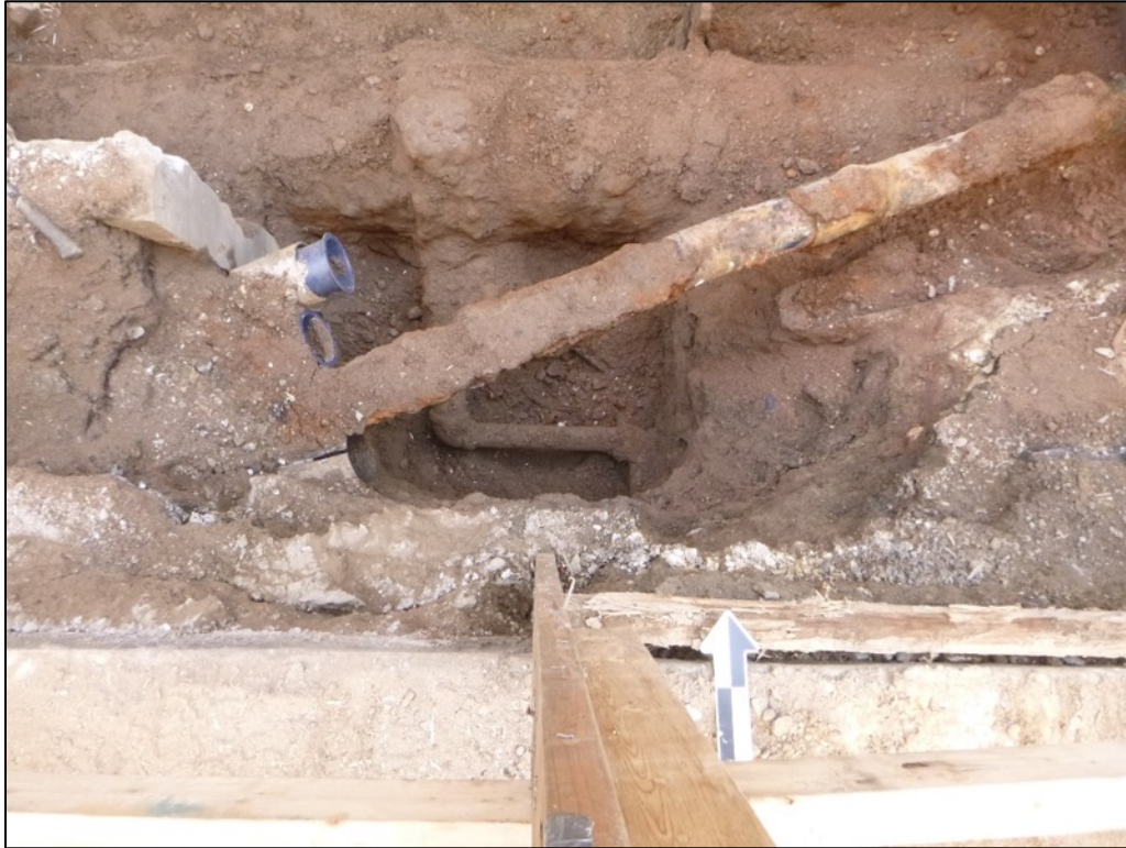
Image 38: Trench 3 Section 3 – Water connection line at 12.1' NAVD88 (5'6" bgs).
