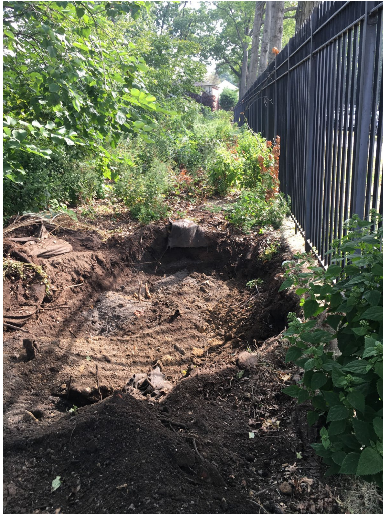
Image 10: Trench 3 excavation to locate existing manhole, facing south.
