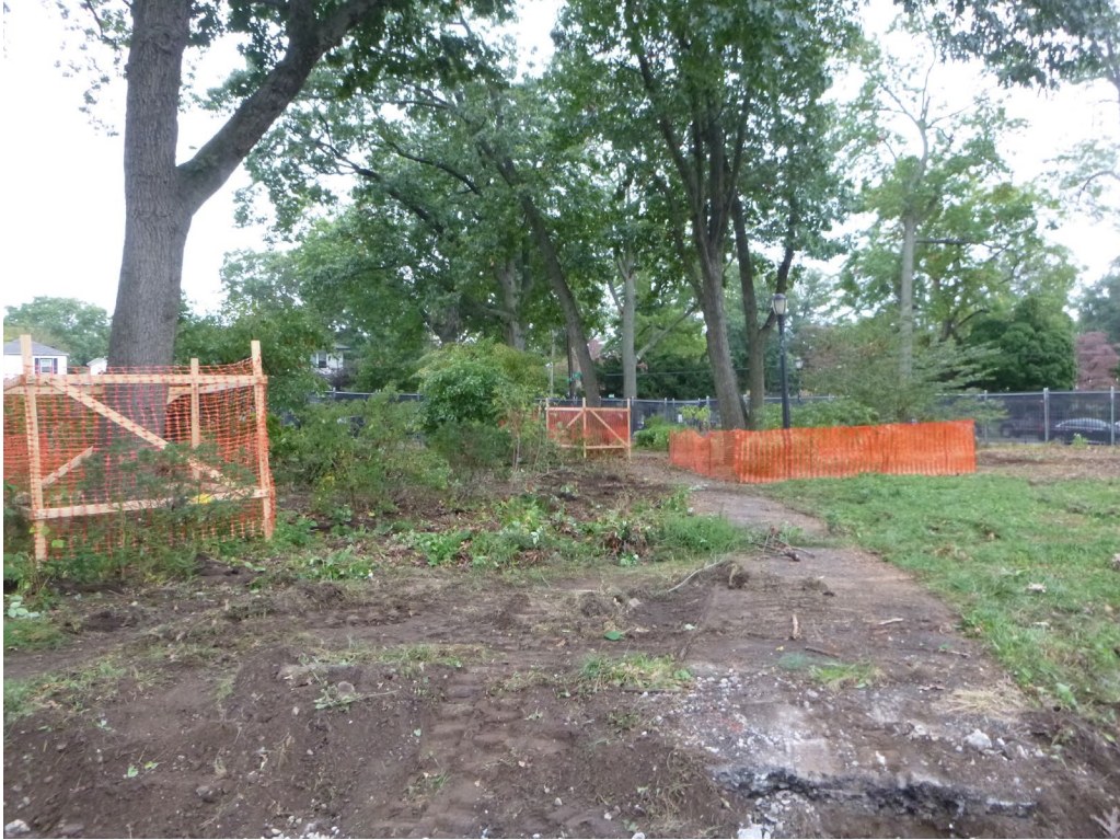
Image 14: Ground surface exposure after grubbing along 165 th Street, facing southeast.
