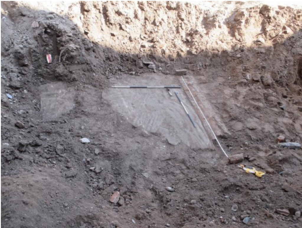
Photo 10 Three-course thick brick wall segment abutting concrete covered bluestone surface/floor identified in AD 1 - AD 2 Trench, also showing the previously installed concrete-encased secondary electric duct bank to the west beneath the marking tape, facing north (Image 3306: May 21, 2021).
