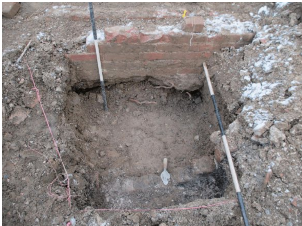
Photo 4 Excavation Unit 2 showing the base of the three-course brick wall on its north side, revealing no spread footer, and the one-course brick wall beneath the trowel, facing south (Image 3698: December 3, 2019).
