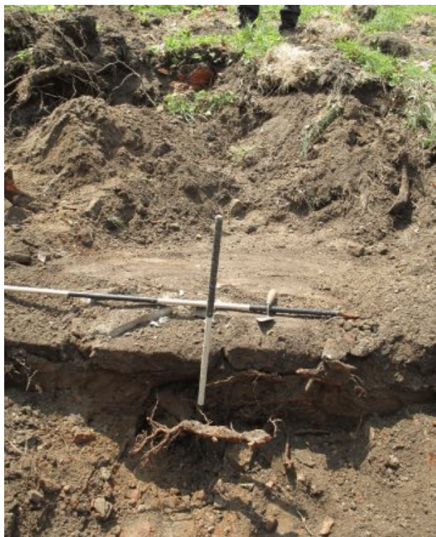
Photo 11 Two layers of concrete surface/floor identified after a large tree was removed in the East Courtyard, facing south (Image 1640: July 9, 2019).
