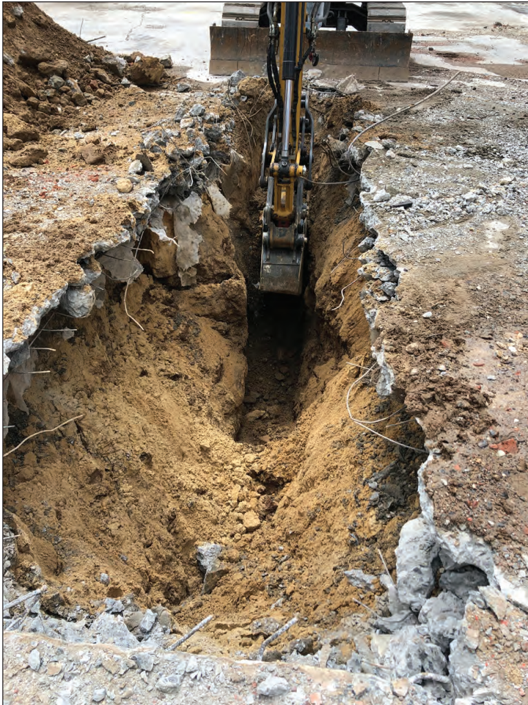
View of excavation of Trench 1; the lighter colored soils in the foreground were the result of the collapse of the trench walls following excavation to greater depths
