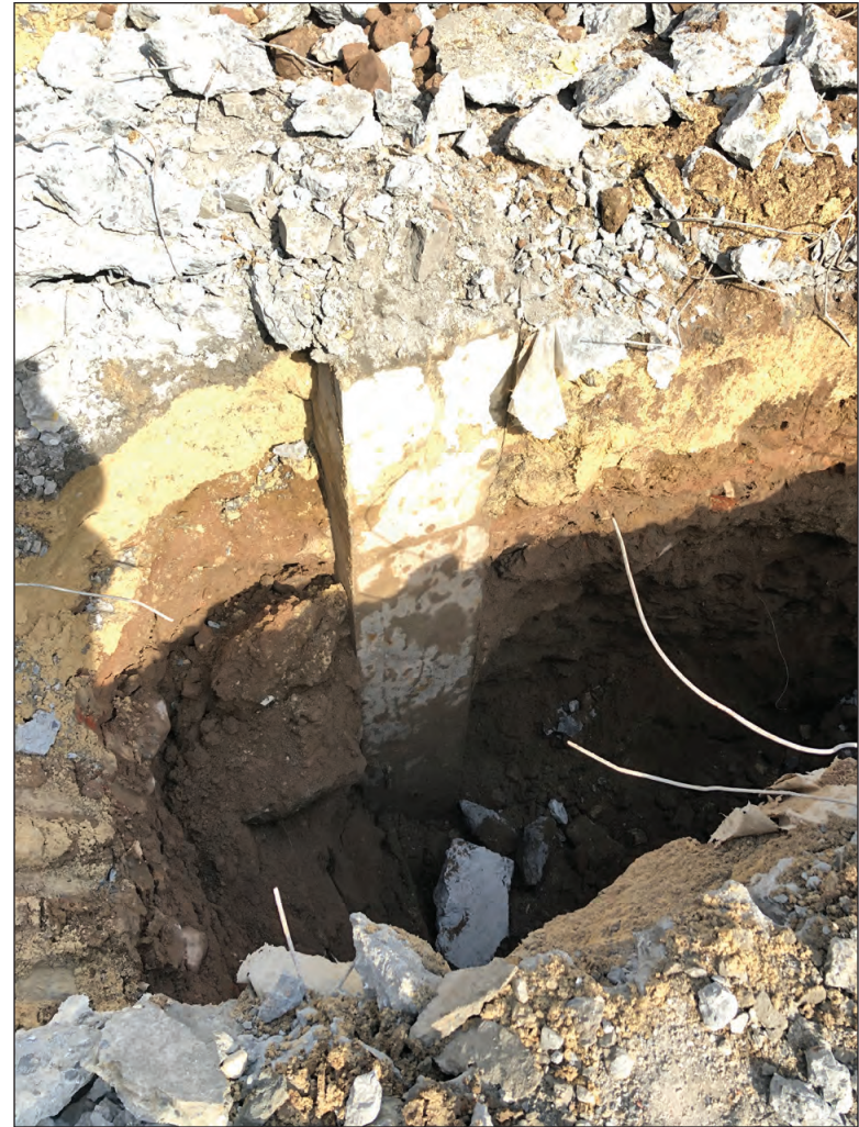
The support column observed within Trench 6 that extended beyond the excavator's maximum reach 12
