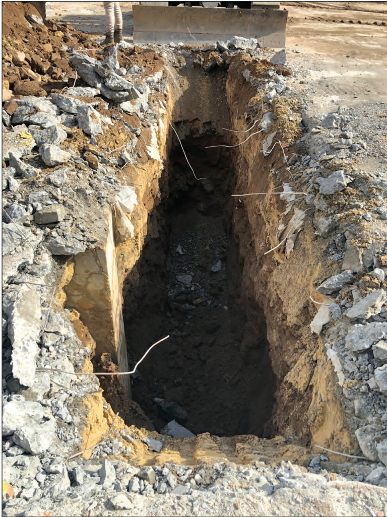
Fill material observed within Trench 6; note column at left 11
