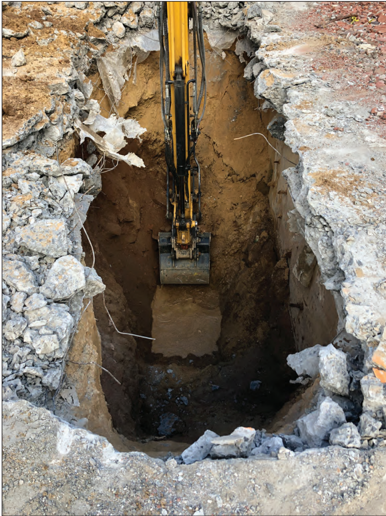
The lowest point of the excavation of Trench 2 where the archaeologists observed what appeared to be subsoil beneath the fill deposit; the backhoe is being used to hold back the soils to prevent collapse
