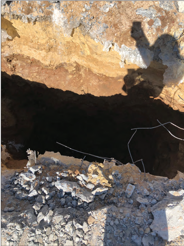
Stratigraphy in the wall of Trench 3, showing the concrete slab, the underlying slab, and the brown fill
