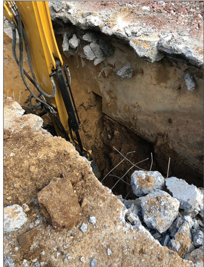
The bottom of the foundation wall observed in the north wall of Trench 2
