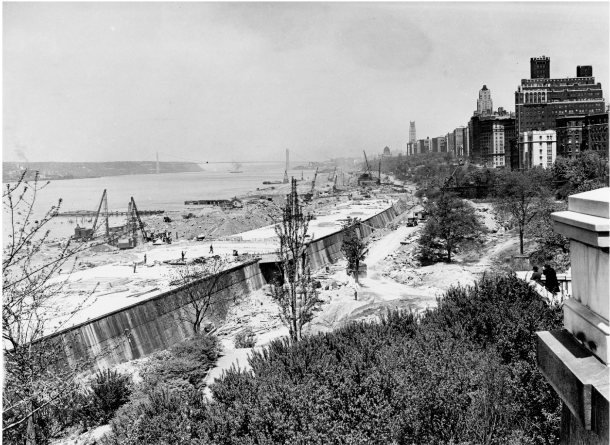
Photo 4. The "train tunnel," or cover, nearing completion c. 1937 (?) with landfill activities underway to the west. The view is north with the George Washington Bridge in the far middle background. (Photo courtesy of M. Bracken (Parks NYC) and N. Catalano (Stantec).
