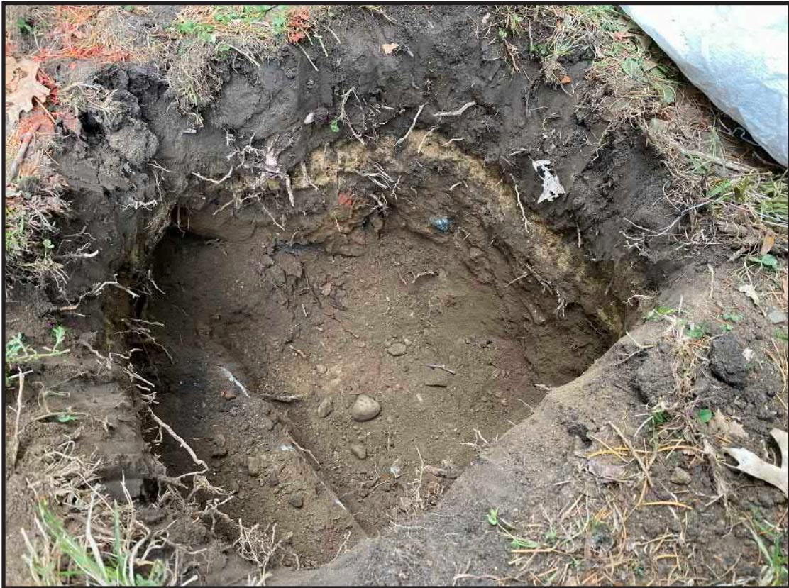
Photograph B.6. Plan view showing the excavation for Sign 15. Note the layer of sand and the edge of a utility vault (Photographer: James Lee, October 2019 [HRI Neg.#19070/D1:016]).
