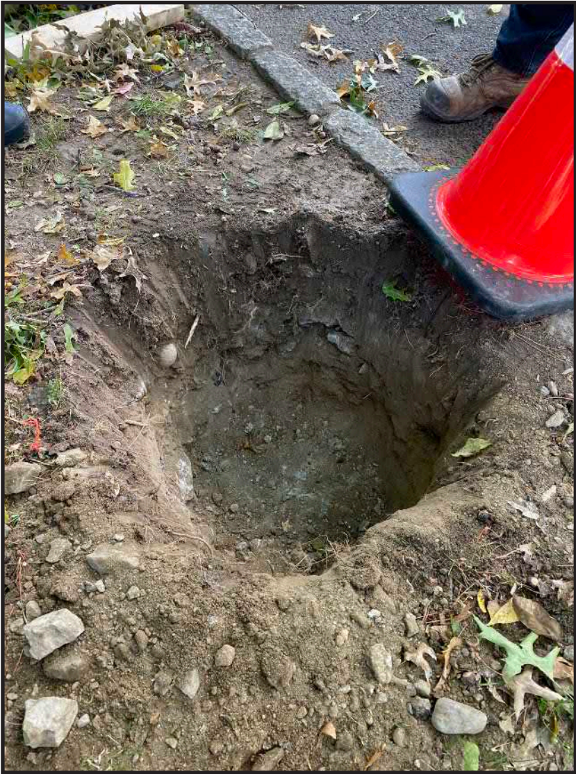
Photograph B.3. View facing northeast showing the excavation for Sign 7. Bedrock was encountered at the base of the excavation (Photographer: James Lee, October 2019 [HRI Neg.#19070/D1:082]).
