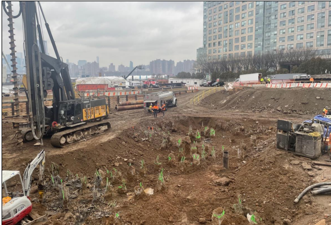
Image 11: A3 excavation area including temporary entrance, facing northwest from Kent Avenue.
