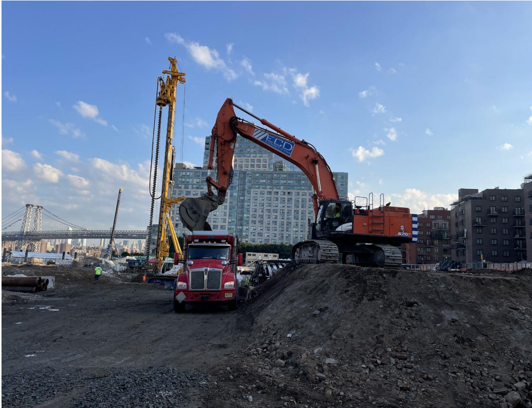
Image 2: Excavation to expose oil storage tanks (Photo courtesy of Tenen, June 2022).
