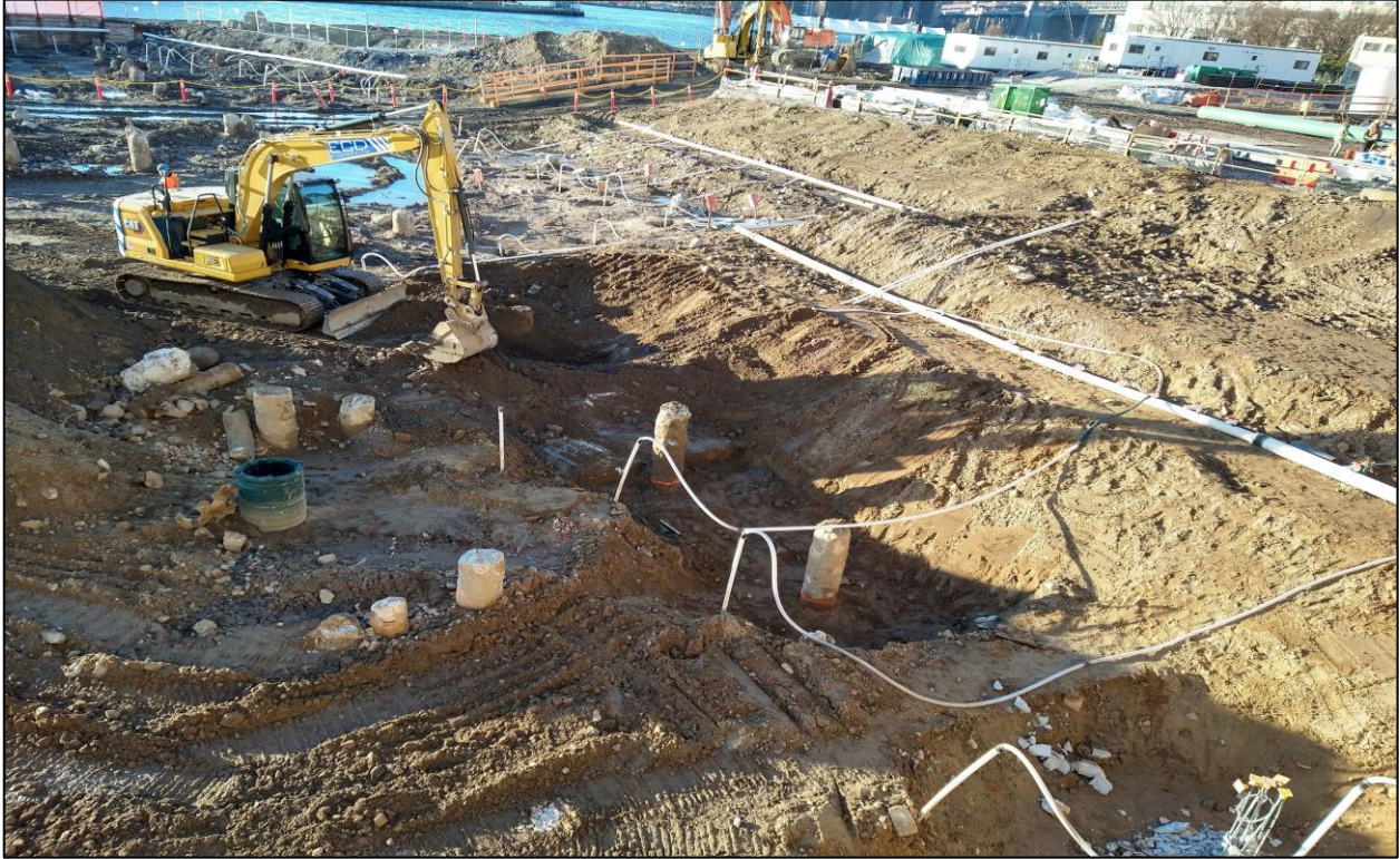
Image 4: View of Areas A1 and A2 from Kent Avenue and S. 11 th Street, looking northwest.
