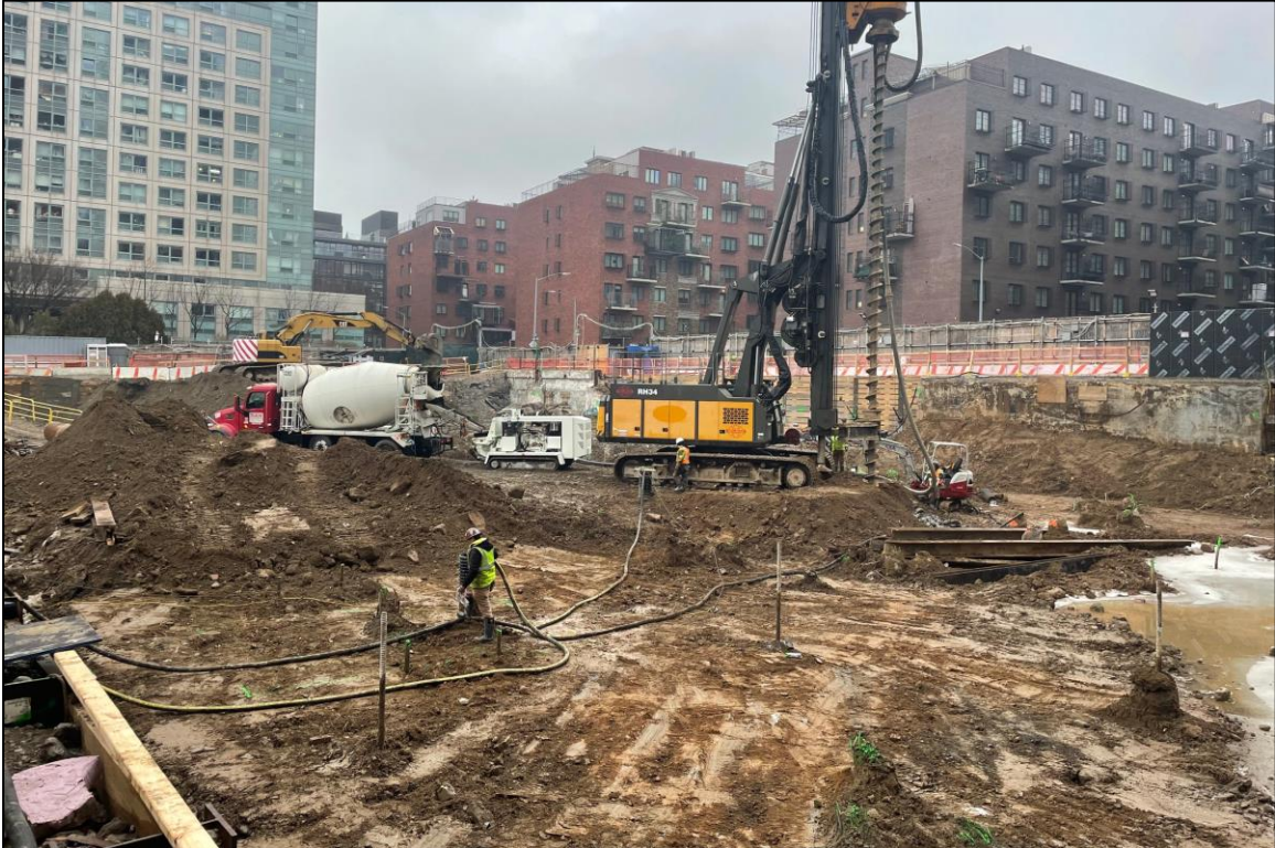
Image 13: A3 excavation area, including spoil heaps and pile driving, facing northeast, standing on ground surface level.
