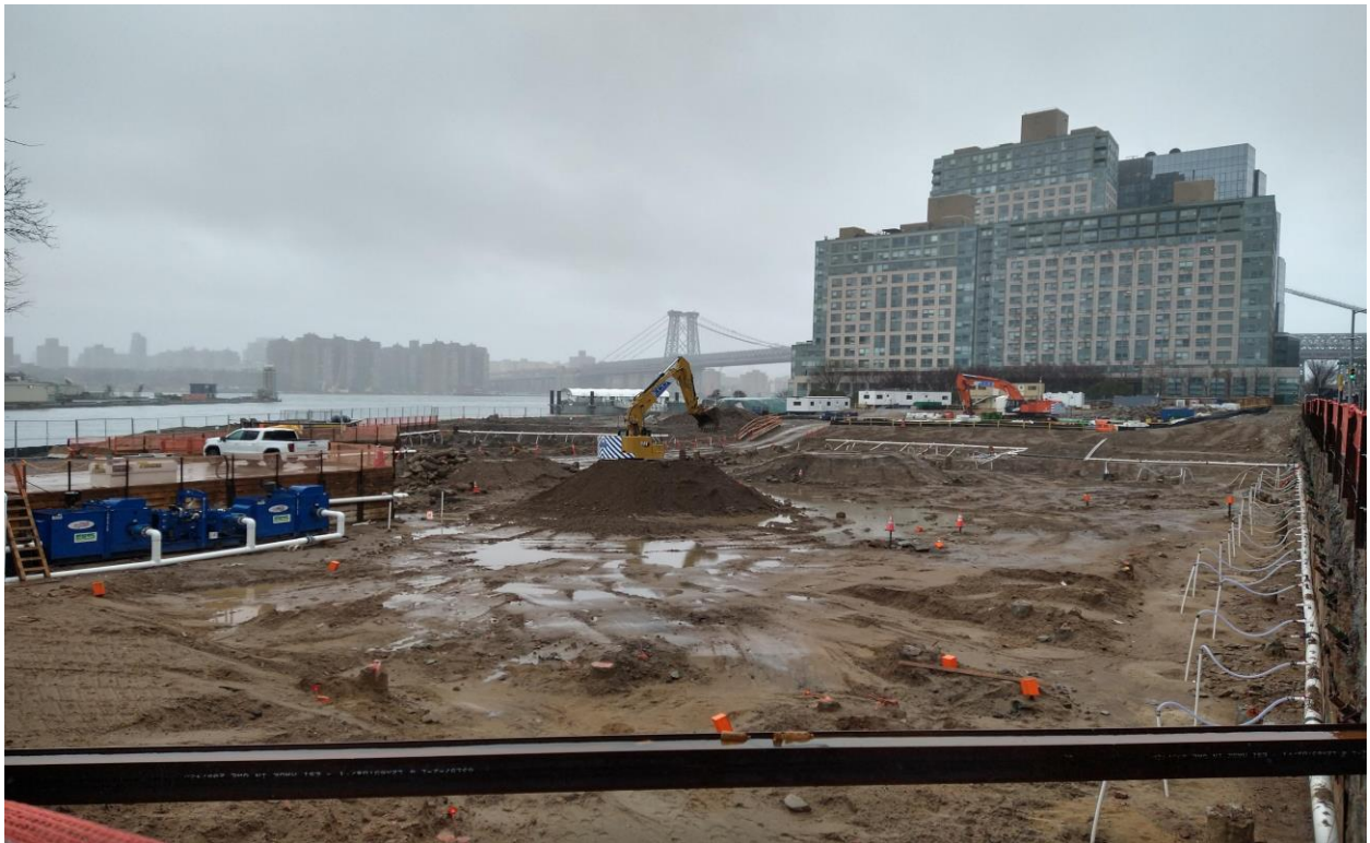
Image 6: Spoil relocation looking northwest from Kent Avenue and Division Avenue.
