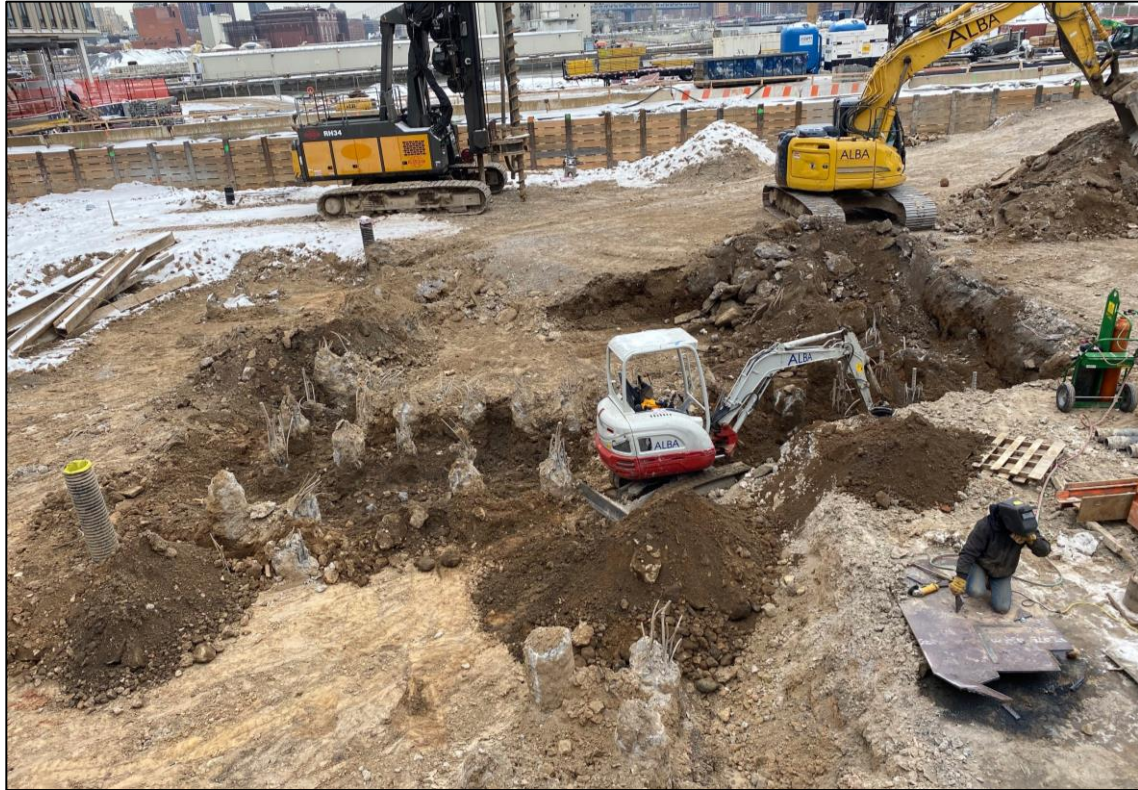
Image 10: Excavation surrounding central piles in A3, view from Kent Avenue, facing west.
