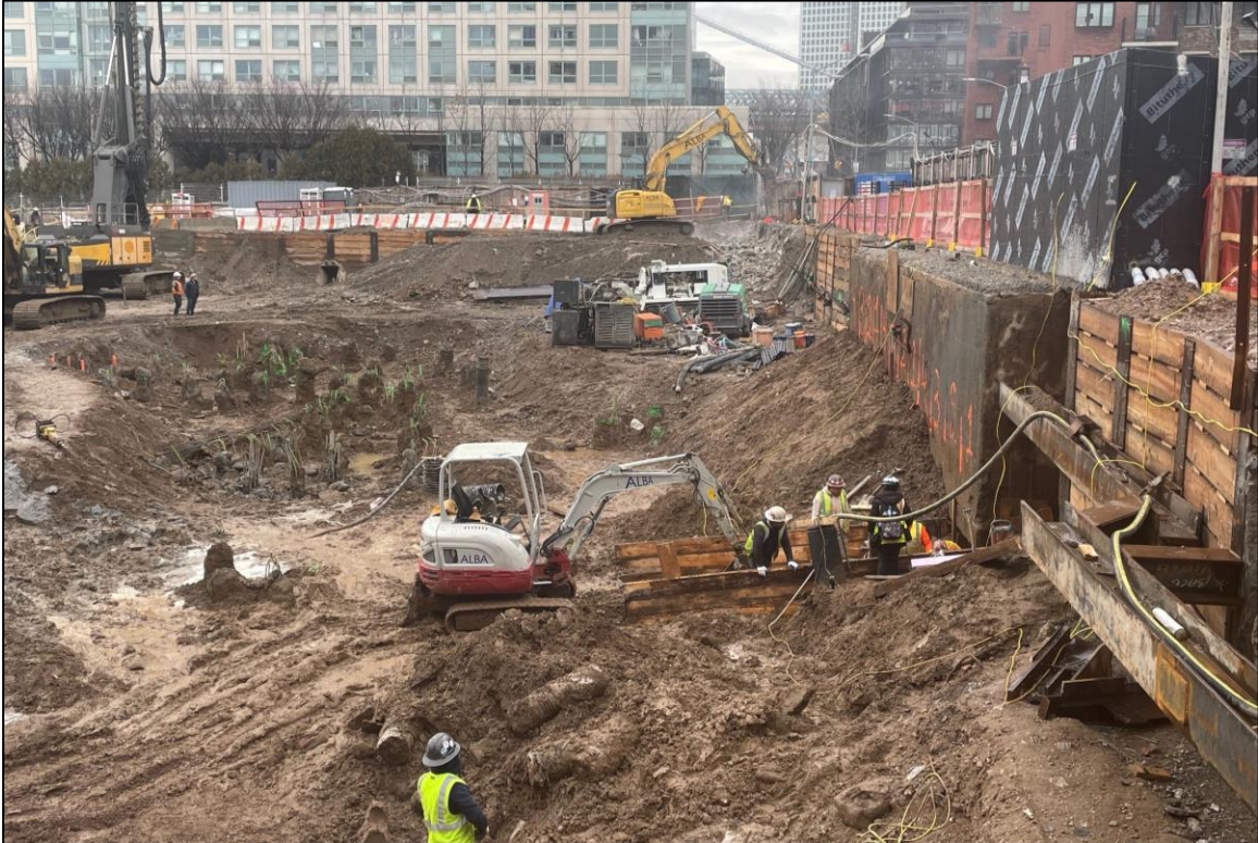
Image 15: View of excavation trench into A3's eastern limit, and existing concrete utility structure along Kent Avenue, facing north.
