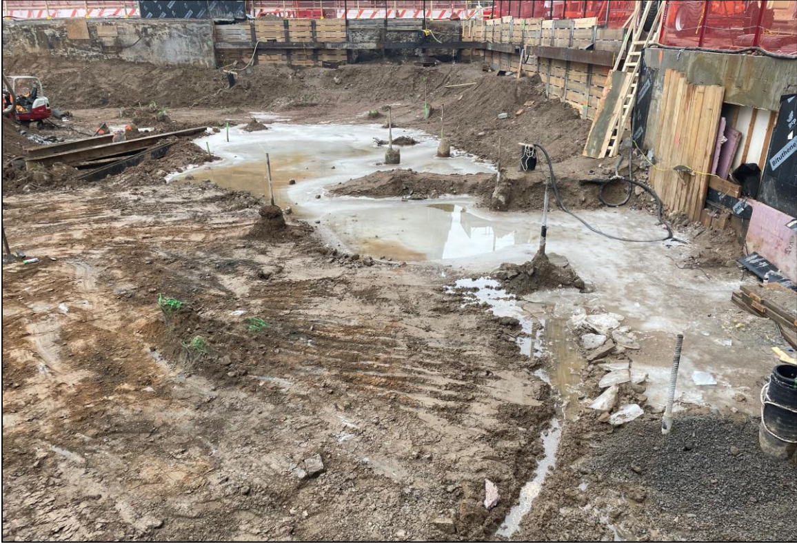
Image 12: A3 flooding mitigation, facing east.
