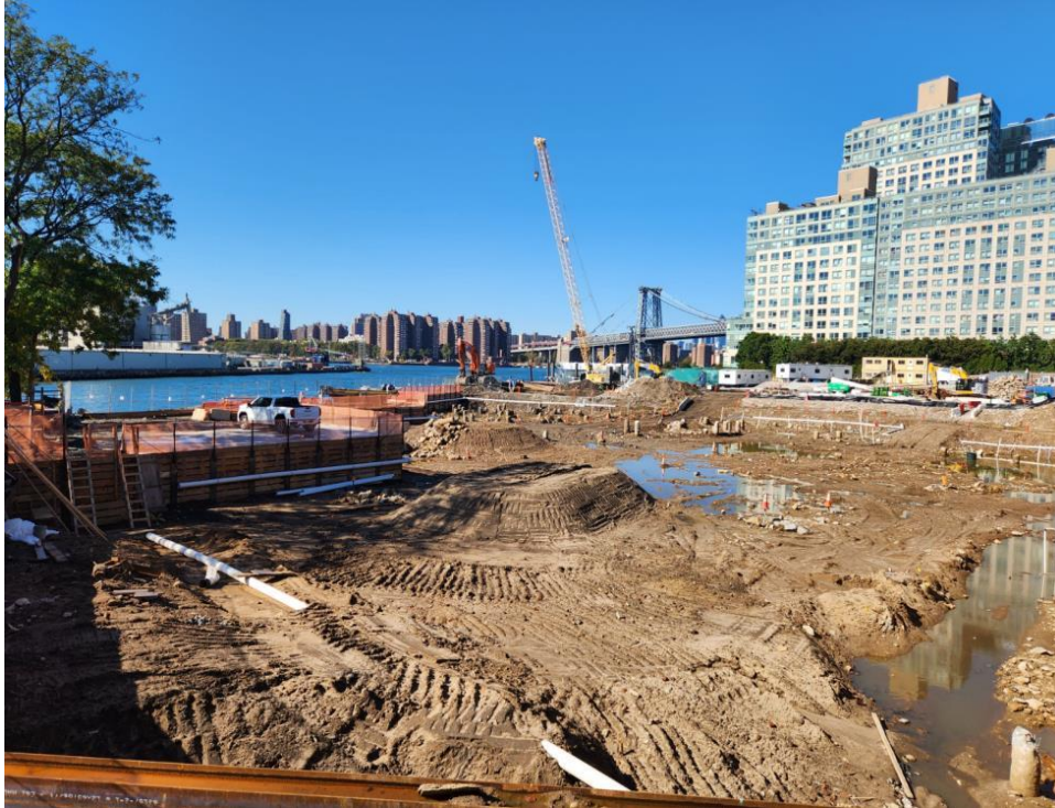
Image 4: Removal of soils from above oil storage tanks (Photo courtesy of Tenen, June 2022).
