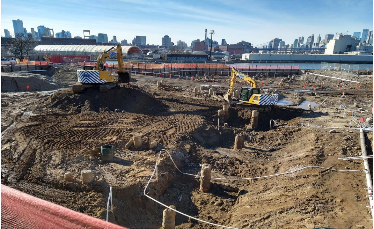
Image 5: Concrete footing slab and cement piles in northeast portion of excavation area, looking west from Kent Avenue and S. 11th Street.
