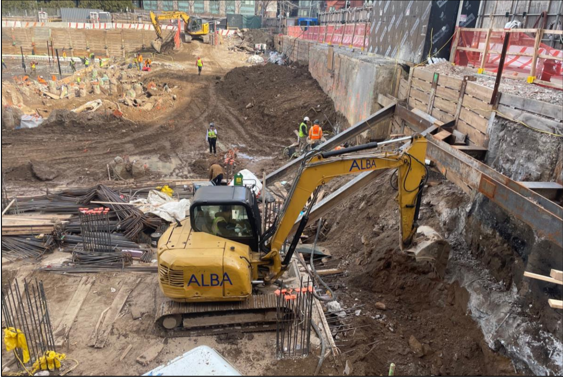
Image 18: Excavation of shoring support, exposing stratigraphy, Area A3, facing north.
