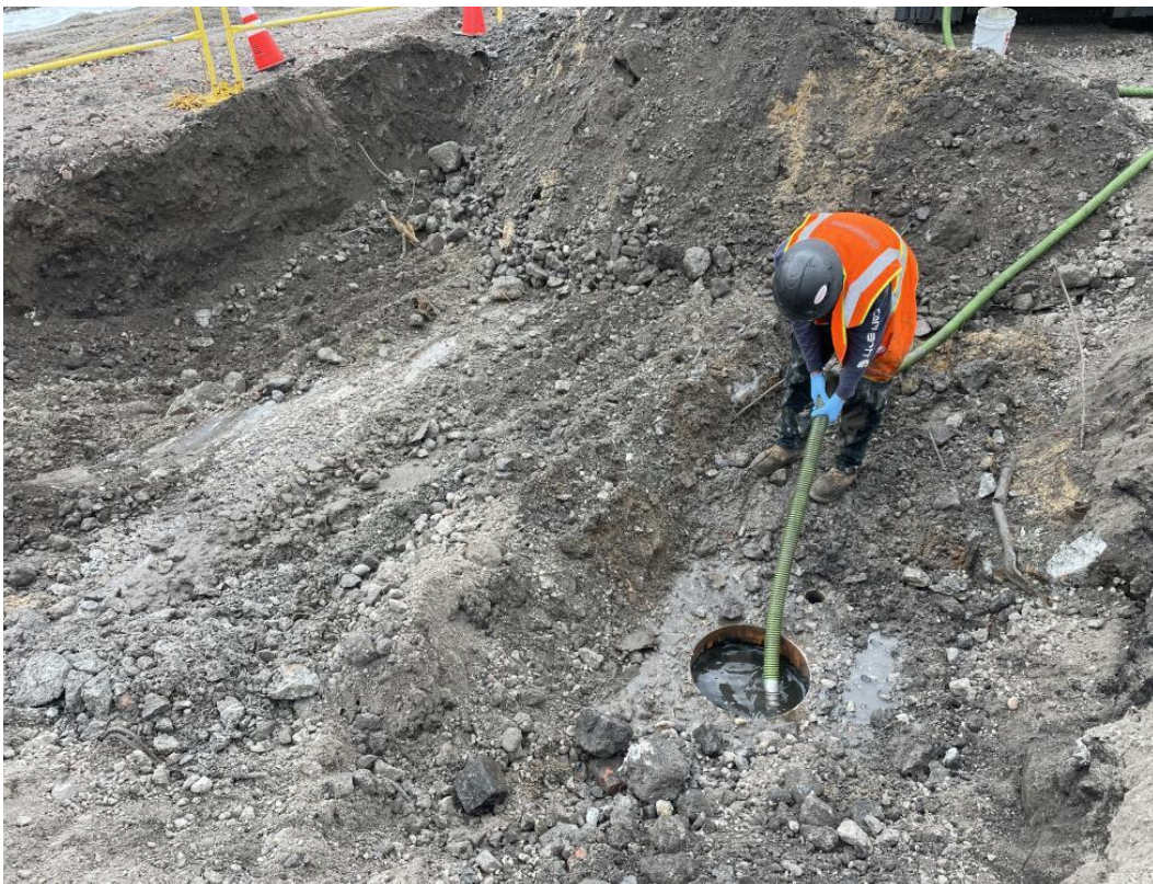
Image 3: Clean-out of existing oil storage tanks (Photo courtesy of Tenen, June 2022).
