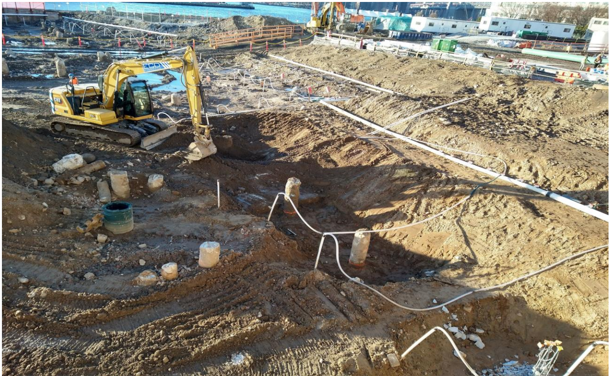
Image 4: View from Kent Avenue and S. 11th Street, looking northwest.
