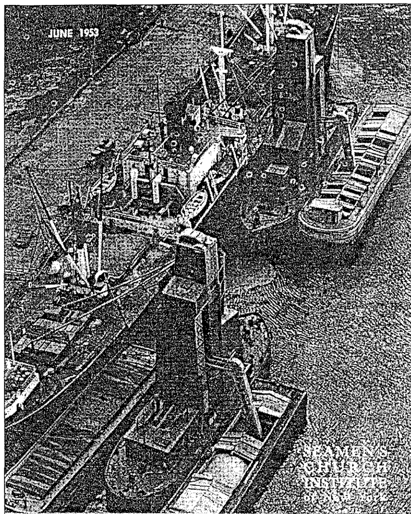
Figure 35. Early 1950s photograph showing two-legged elevators. Note the “skyscraper on a tugboat” look of these vessels, as well as the canal boats and hold barges offloading their cargos of grain (as presented in Baab 1953).
