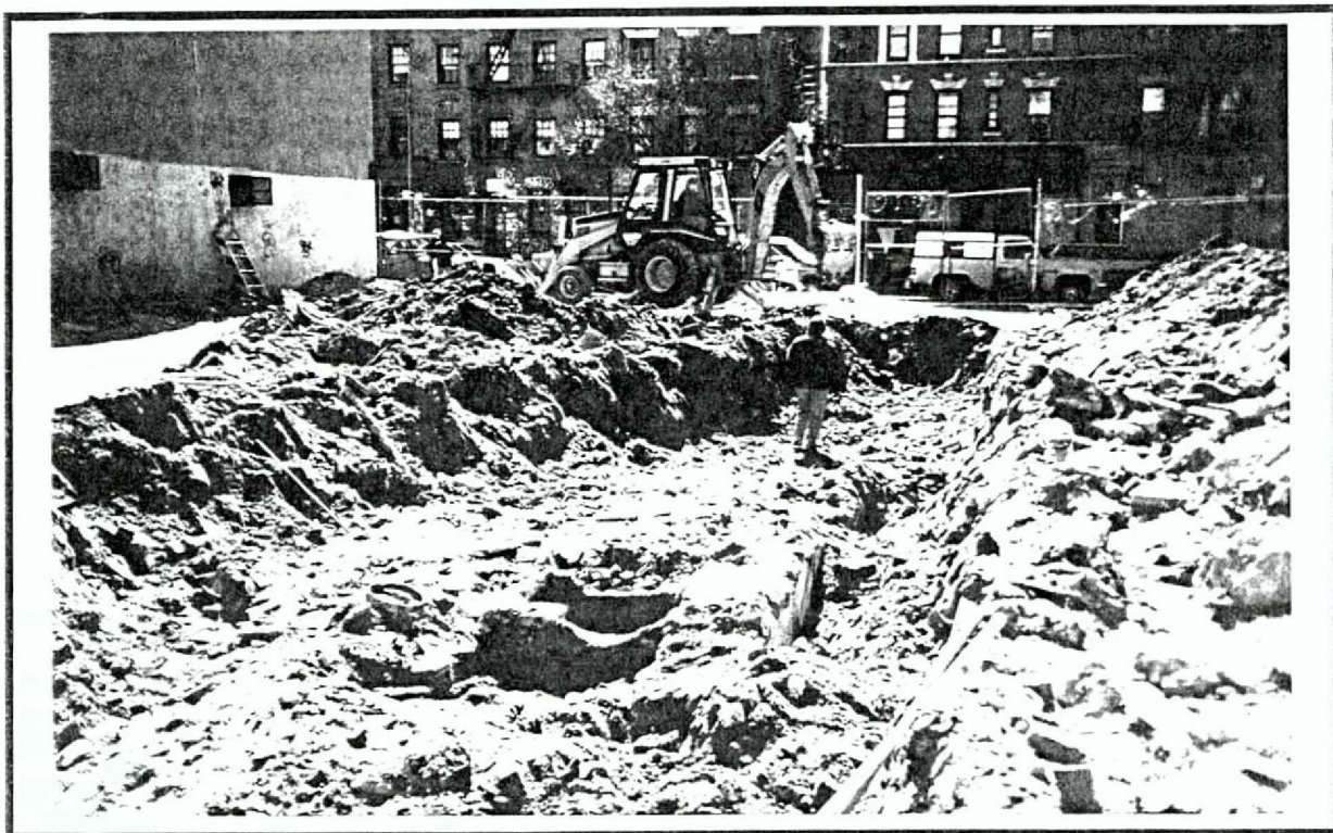
Photo 7: In an effort to locate any subsurface features 100% of the testable area was exposed by the backhoe.
