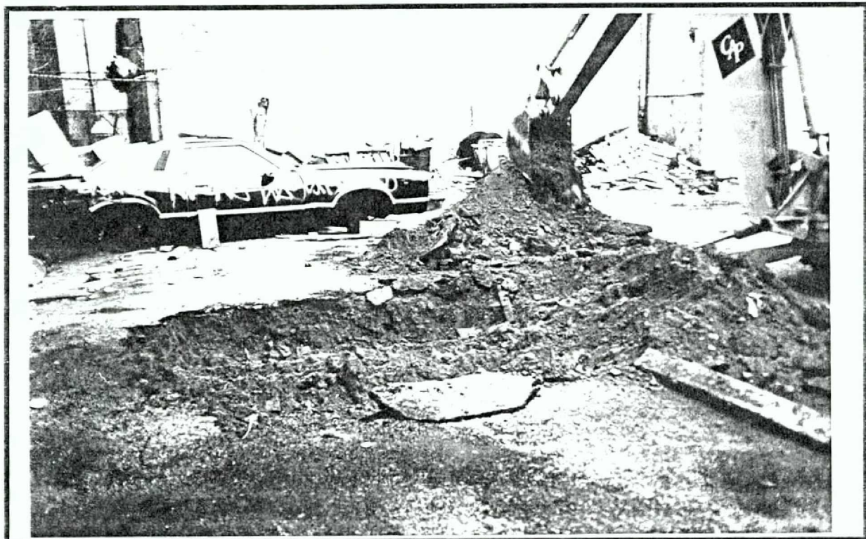
Photo 4: Backhoe carefully removed asphalt paving and layer of fill to determine level of overburden. Yellow/orange sandy gravel represented fill on which paving was laid.
