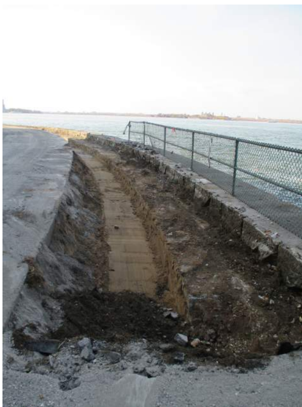
Photo 18 The completed seawall repair excavation from Stations 10+23 to 10+88 showing the concrete seawall buttress, facing south (Image 3639: October 29, 2013).
