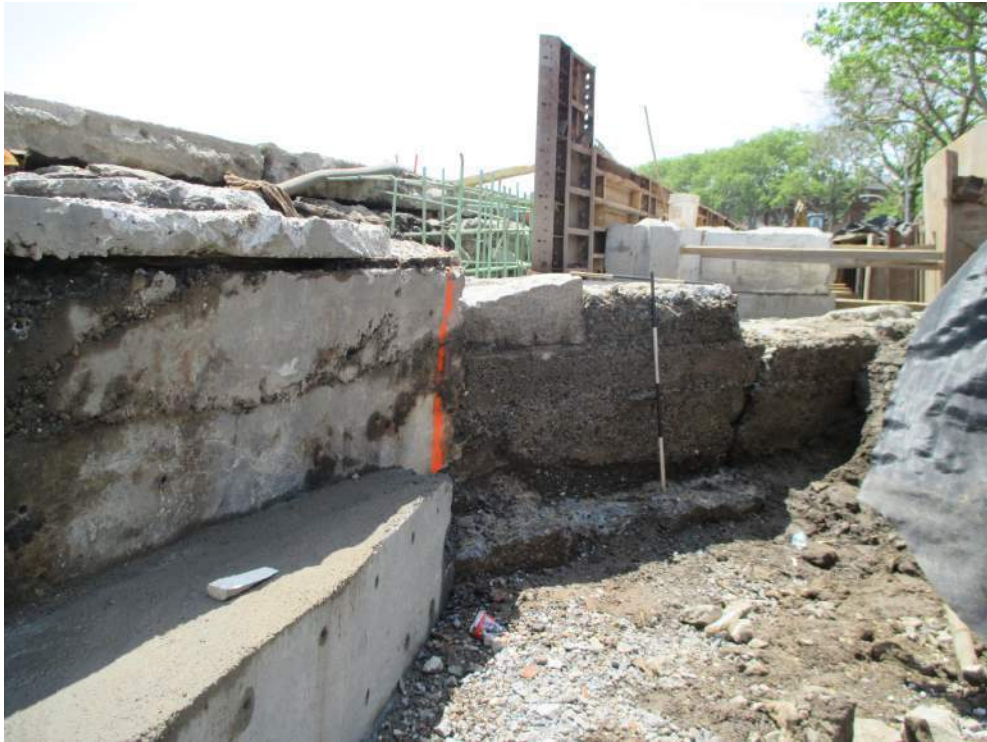
Photo 3 The landward side face of Feature 3, the 1883 seawall, within the seawall repair excavation showing more recent repairs to the left (east), facing southeast (Image 4558: June 30, 2014).
