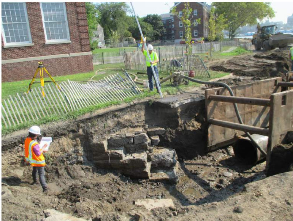
Photo 4 The portion of the storm drainage trench between CB 10.01 and MH 10.05 showing part of the waterside face of Feature 3, the 1883 seawall, facing northeast (Image 5185: August 8, 2014).
