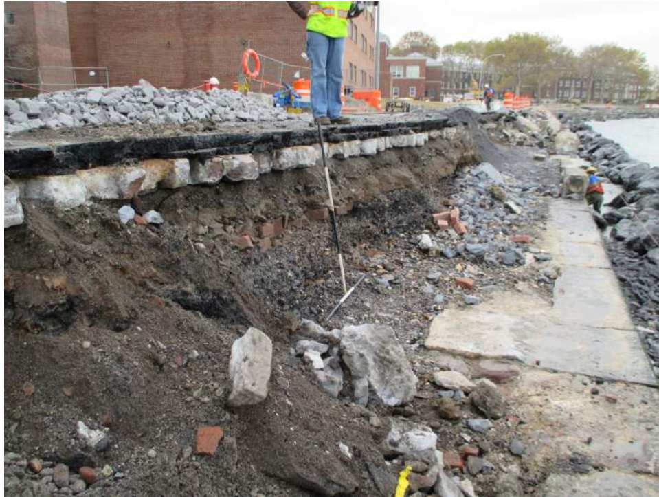
Photo 19 Excavation for the seawall repair around Castle Williams showing the stratigraphy beneath Carder Road, from near Station 13+20, facing south (Image 3522: October 16, 2013).
