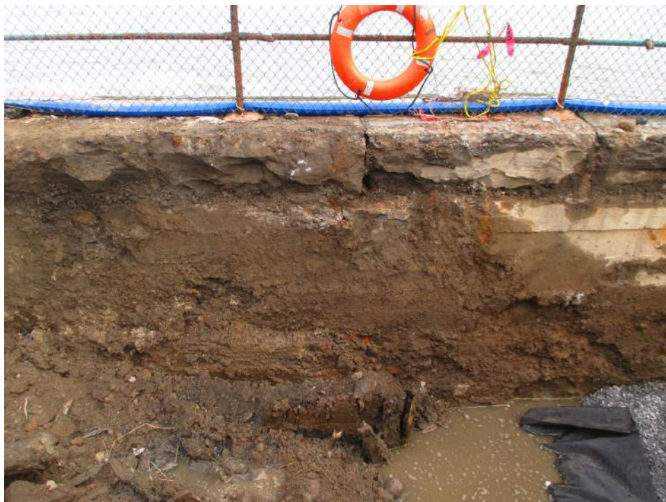
Photo 20 Seawall repair excavation in progress from Stations 9+50 to 9+60 showing remnants of the wooden forms used during seawall construction at the base of excavation, facing north (Image 4204: April 17, 2014).
