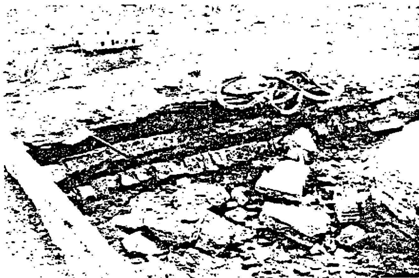
Plate 7. Stratified layers of pavement. Surface and middle layers are concrete and bottom is Belgian block. Each has a base of about 30 cm. of cinders.
