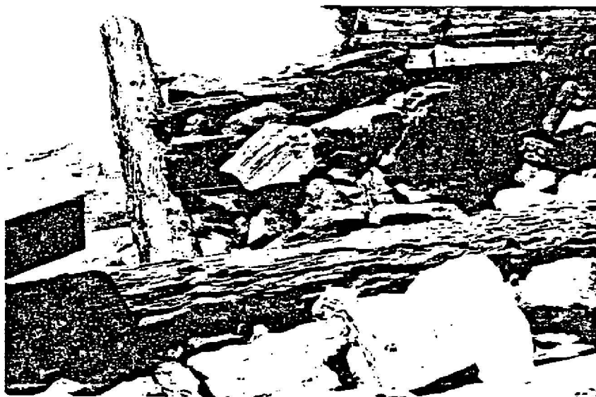
Plate 12. Another view of station 122+00. Note the logs used for cribbing and the stone ballast.
