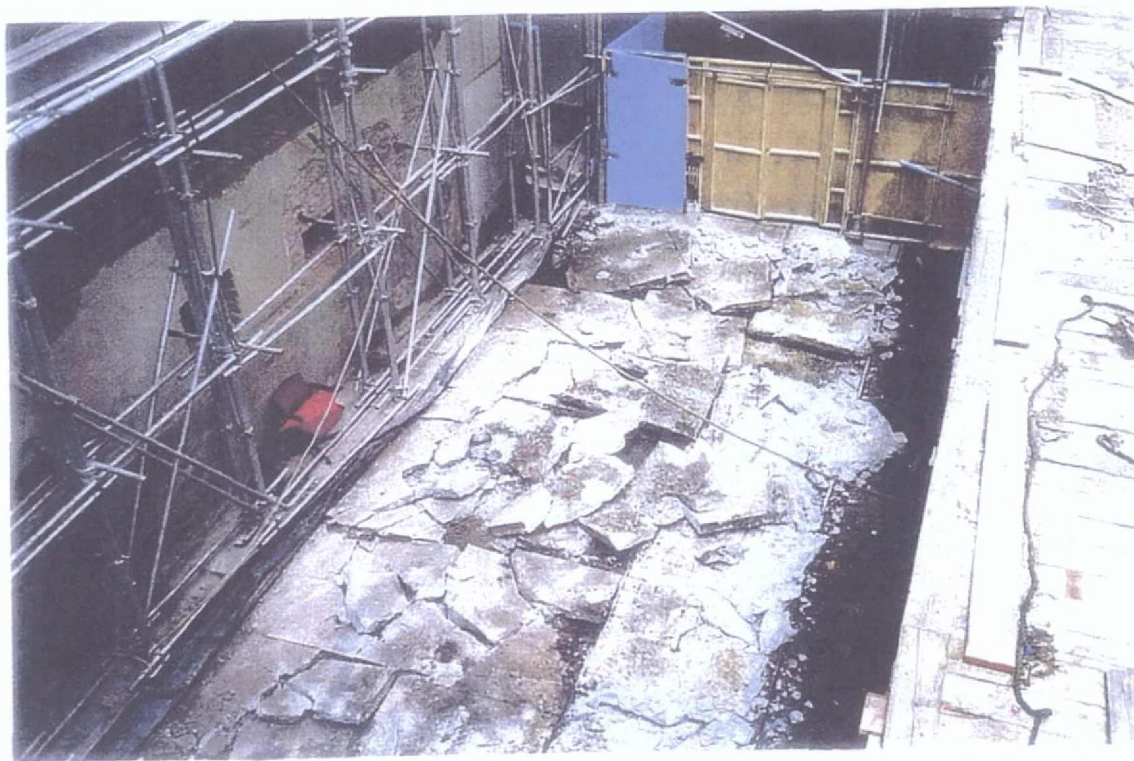
Fig. 2. View of the project site looking east: removal of the sidewalk and street pavement.
