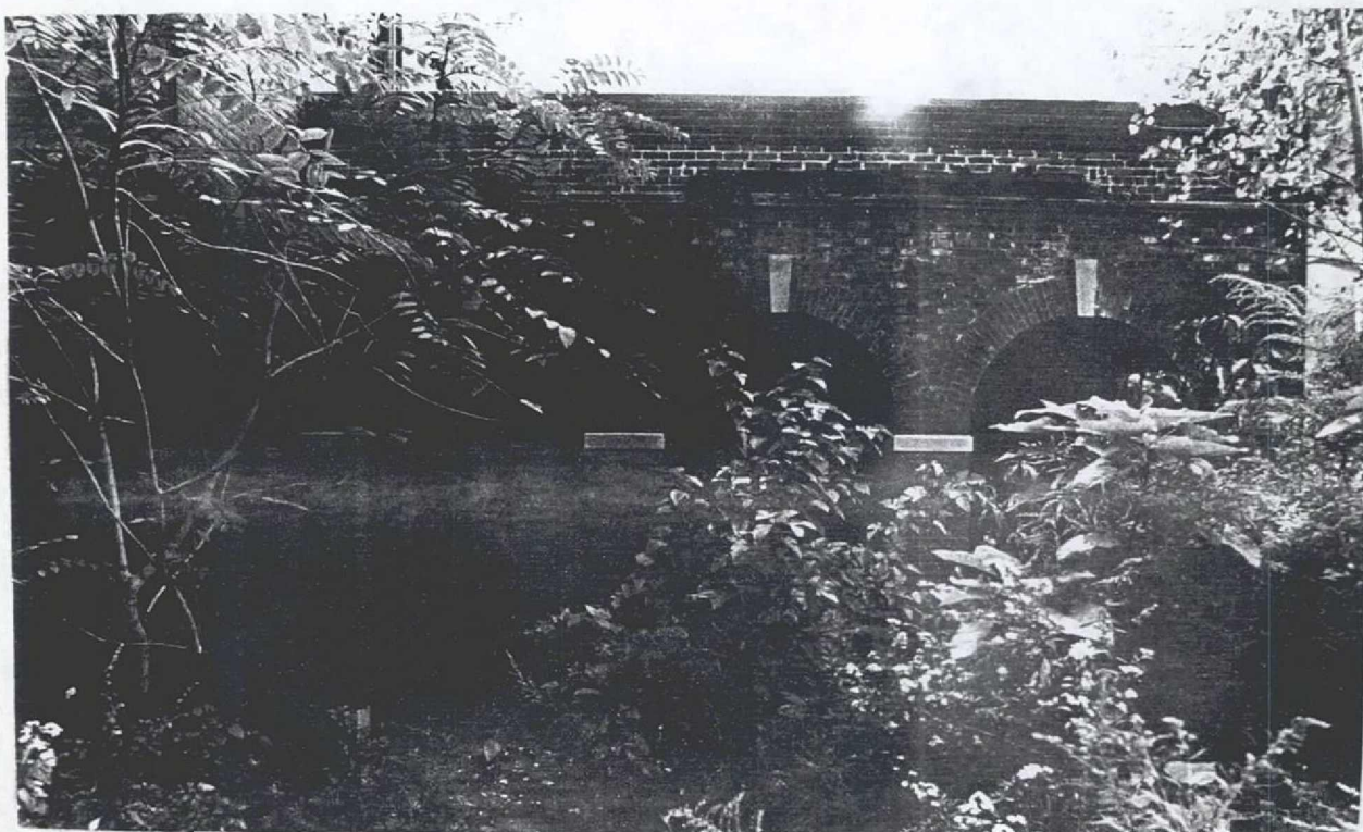
FIGURE 19. Detail of the loading dock section of the Bakery Building showing brick arch openings with limestone keystones. (Michael Spozarsky, photographer, Oct. 1980)
