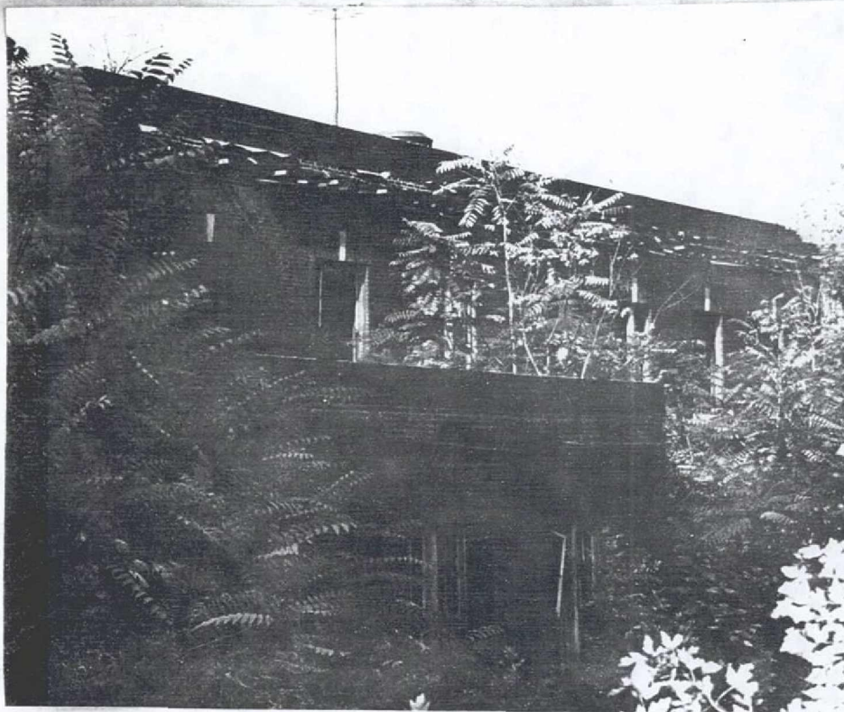
FIGURE 20. East facade of the Bakery Building. Note the deteriorated wooden cornices just below the parapets. (Michael Spozarsky, photographer, Oct. 1980)
