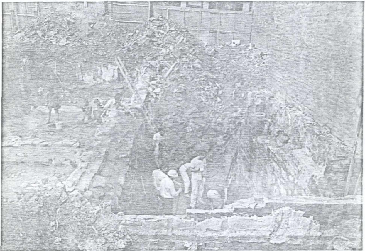
FIGURE 46. Photograph of Lots 24 (left) and 25 (right) (69 and 71 Pine Street, respectively) during the removal of the concrete floor from the rear, southern portion of Lot 25. Note the higher elevation of the basement floor in Lot 24 to the west. Also, note the common or party foundation wall separating the northern parts of the lots, versus the separate foundations for later (southern) additions. View is to the north. (Photographer: Tony Masso, 1984).
