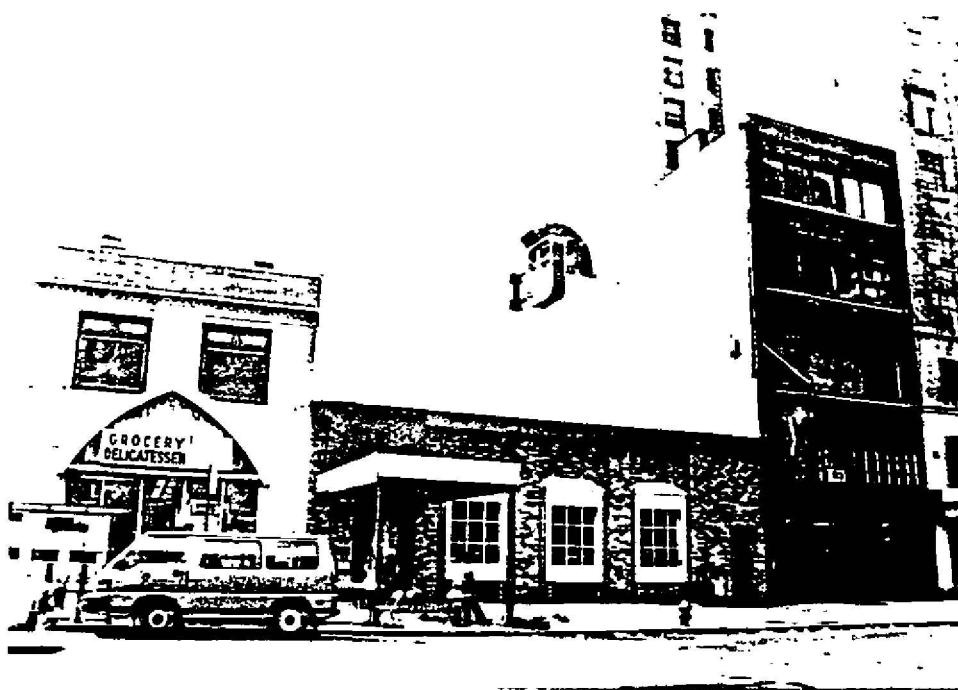
Photo 6 Area A, Lots 47 (left two bldgs.) 52 (5-story bldg.), south side of 23rd Street, looking south.
