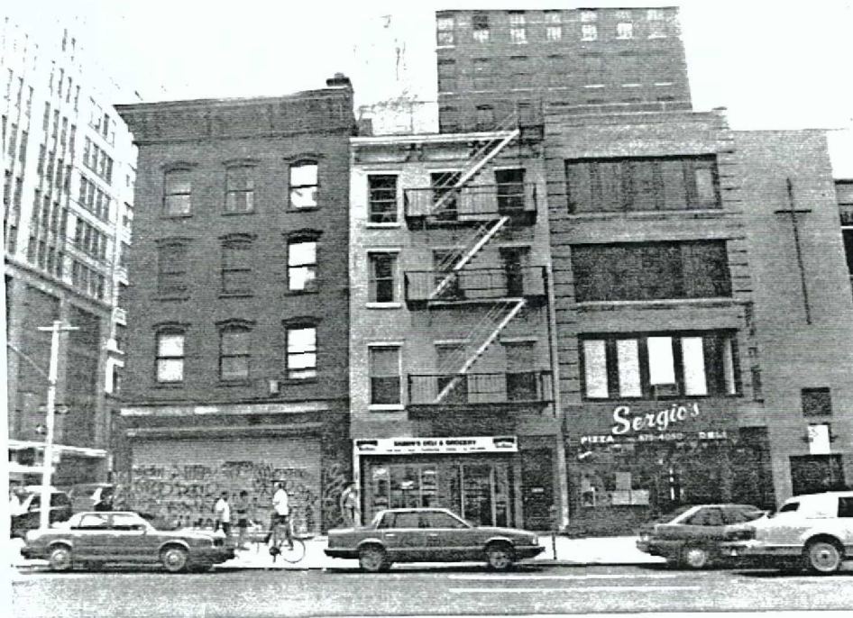
Photo 4: 261-255 Seventh Ave., Lots 77,78,79 from west.
