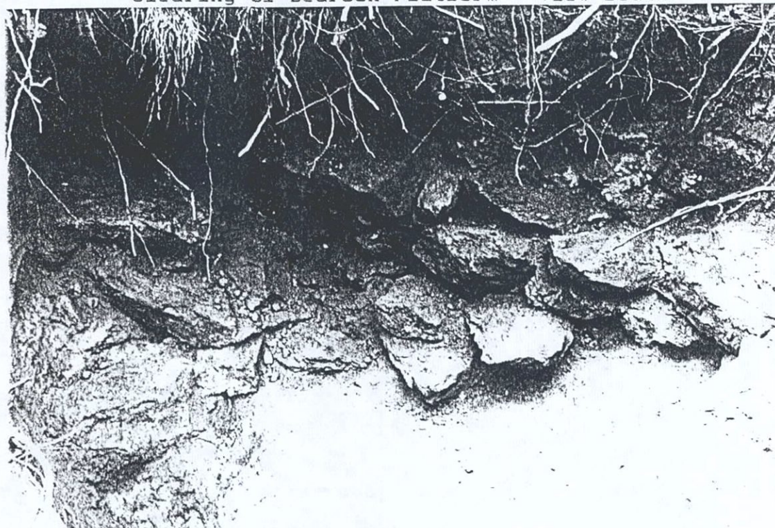
Plate 41 Western Dry Well Excavation Detail - Dry Laid Stone Retaining Wall in Southwest Corner of Excavation View South
