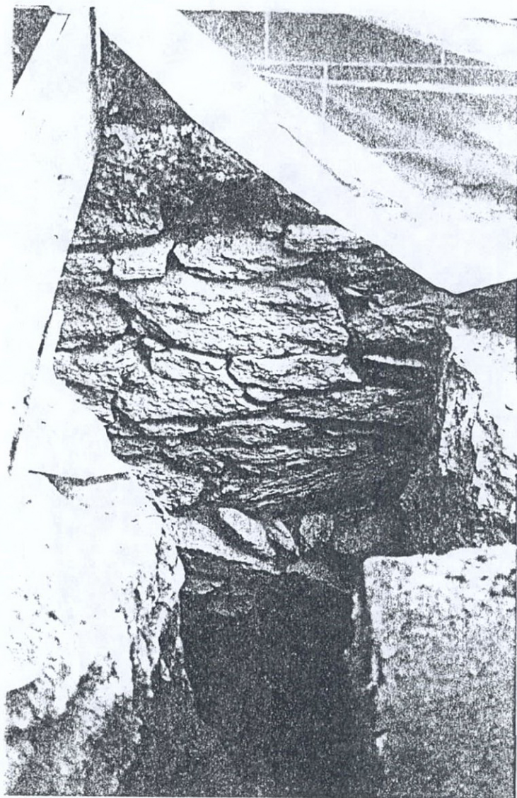
Plate 24 Northwest Mansion Foundation Wall Portion Immediately East of Areaway View North
