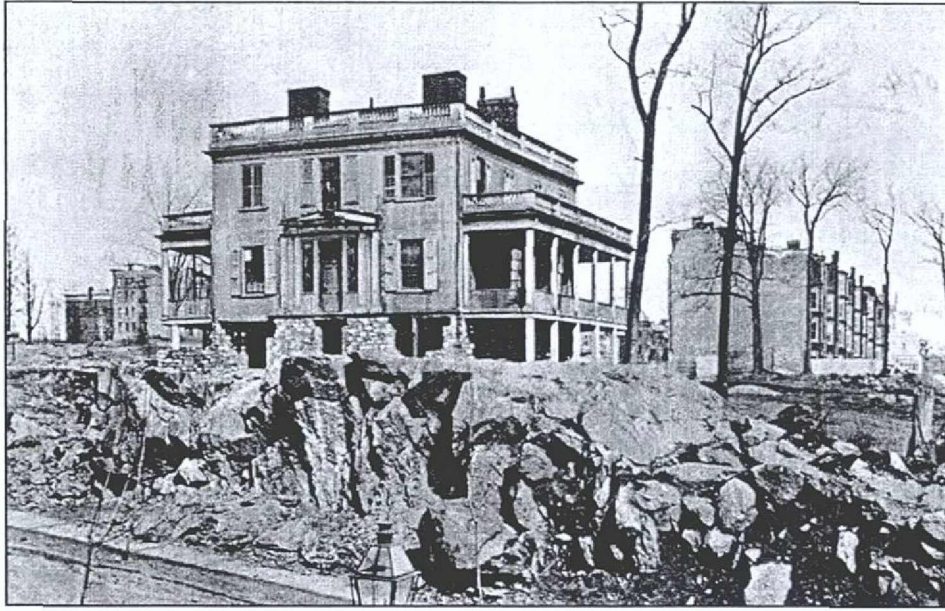
Figure 5-10. Photograph of Hamilton Grange during its relocation, view north, ca. 1889 (source: LOC 2003b).
