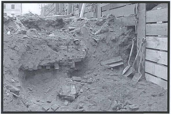
Plate 2.2 Lagging Wall and Tieback Support System for Southern Boundary of Project Area, View Looking Southwest.
