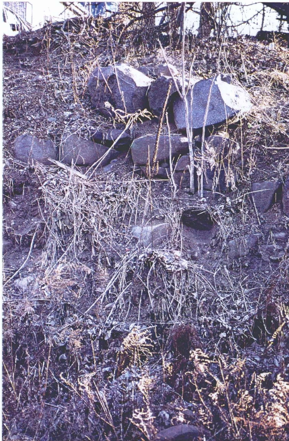
Figure 20 Detail of the eastern embankment showing the partially exposed section of the unmortared stone retaining wall.
