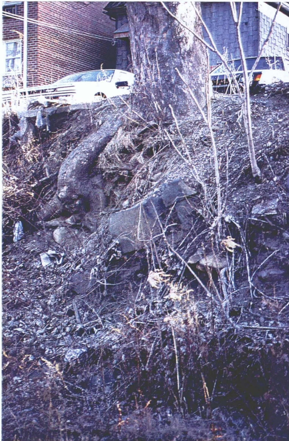
Figure 21 Detail of the eastern embankment showing the exposed root system of a large tree along the edge of the property, which indicates that the original cutting and grading operations were more recent than the age of what appears to be a 20th century tree.
