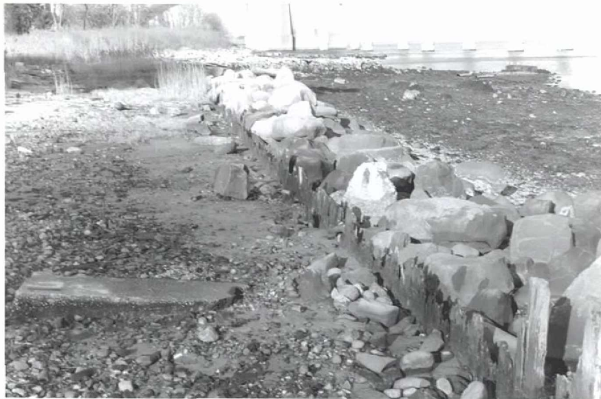
Plate 7 Remains of Wooden Bulkhead and Rip-Rap Block 4602, Lot 50 View North
