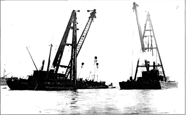
Figure 8. Undated photograph of two A-frame crane barges involved in what appears to be a salvage operation. Note scow hulls, the machinery cabin, as well as the numerous crane stays on the barge to the left. These stays and their corresponding chain plates where they attach to the hull are a distinguishing characteristic of this vessel type (courtesy of the South Street Seaport Museum).
