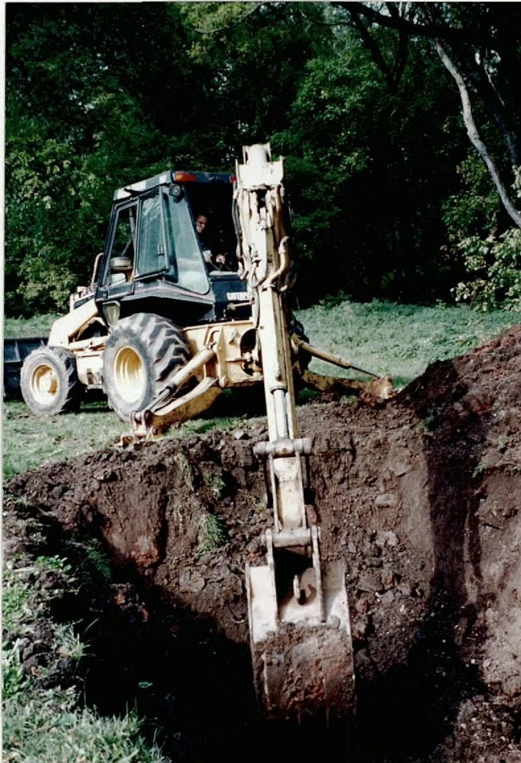
View of Mill Pond project excavations in progress
