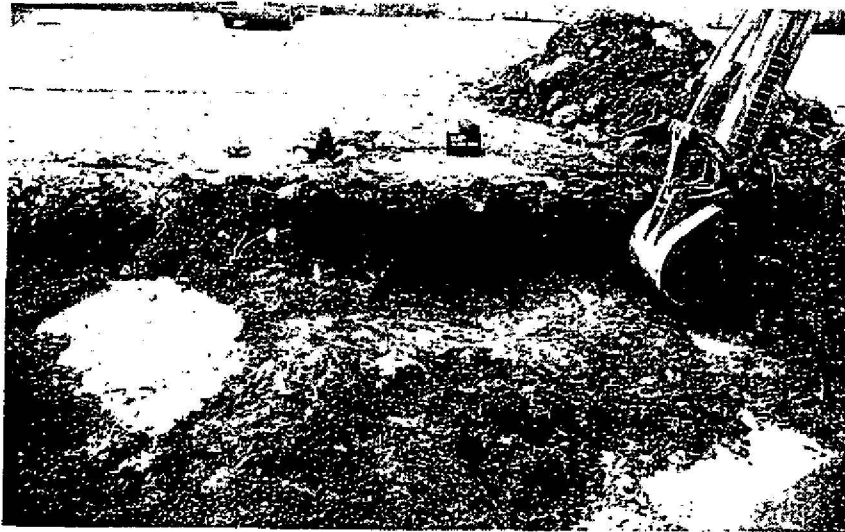
12 Test Area G1 Pit 4. View is looking south across the pit. A small section of stone (arrow) that may be a foundation of some sort is cut into the shallow rock outcrop or bedrock and apparently extends under the pavement to the south. Note water on the left seeping into the excavation. (photo Geismar 3/10/93)
