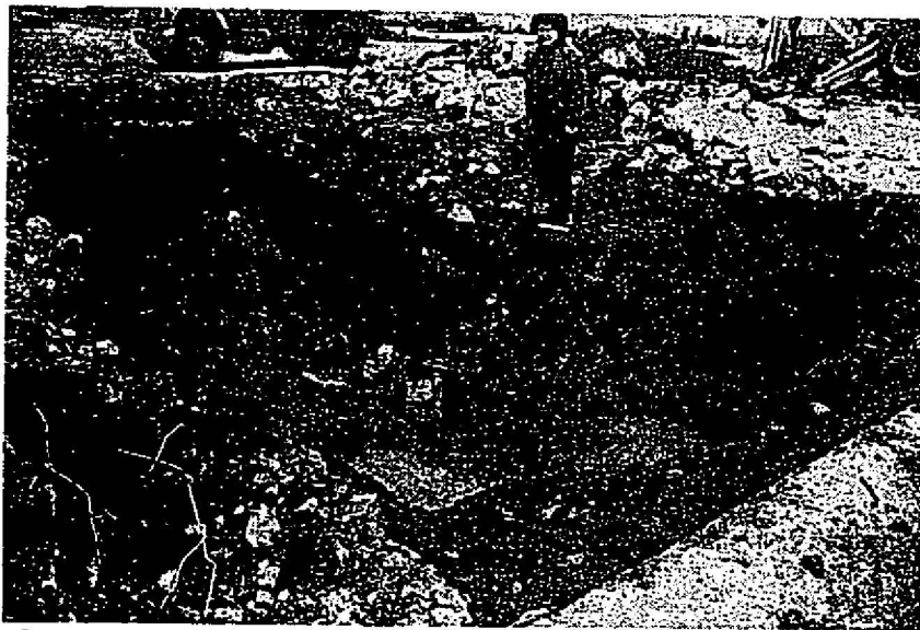
6 Test Area G1 Pit 1 at the end of excavation; the view is to the southeast. Note water in the bottom of the pit and tumbled boulders. Bedrock and outcrops seen in the excavation are now obscured by the water. (photo Geismar 2/11/93)
