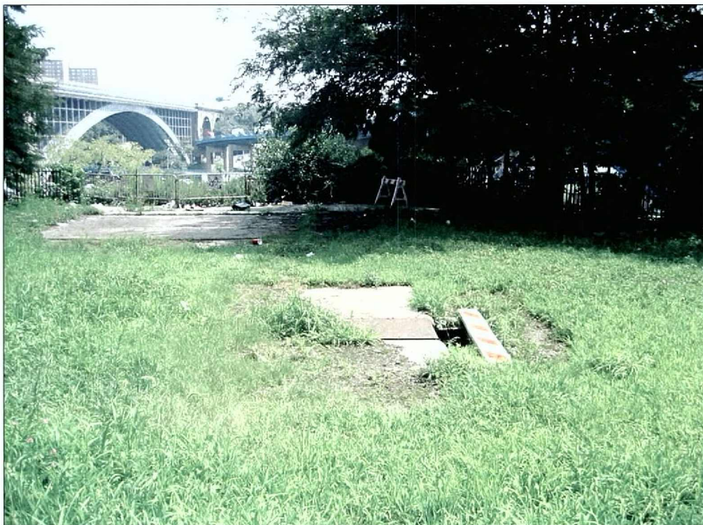
Photo 3-3 Looking east from within footprint of former Shaft No. 25 Gate House. Note rectangular opening in foreground that provides access to subsurface remains, and concrete slabs atop pump shaft in background.
