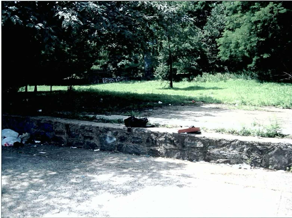
Photo 3-2 Looking west from overlook area on Shaft House No. 25 and Blow-Off Vault roof. Note cut-stone curb and concrete slabs beyond curb that rest atop the pump shaft. Former Shaft No. 25 Gate House was located west of the curb.
