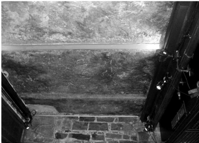
**11** Underside of the sidewalk exposed adjacent to the brick street vault seen in Figure 10. Here, too, steel beams were introduced to support the vault. Note the mortared stones of the end wall of the vault. (Geismar 5/19/05)
