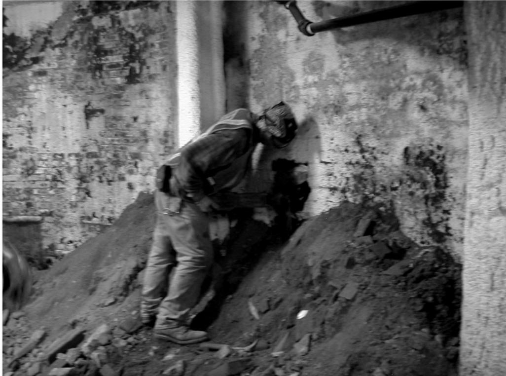
**3** Construction worker attempting to determine the thickness of the basement wall of 170 Broadway. The attempt was ultimately abandoned when it became apparent that the wall was more than a brick facing to the wall exposed on the south side of the Maiden Lane utility trench. (Geismar 5/9/05)
