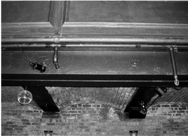
**10** Brick street vault, an extension of the basement in the City Hall Restaurant on Duane Street. The vault's arch, which runs perpendicular to a brick street wall, is shored by iron beams. The long steel beam seen in the upper foreground replaced cast-iron columns that originally supported the structure. (Geismar 5/19/05).
