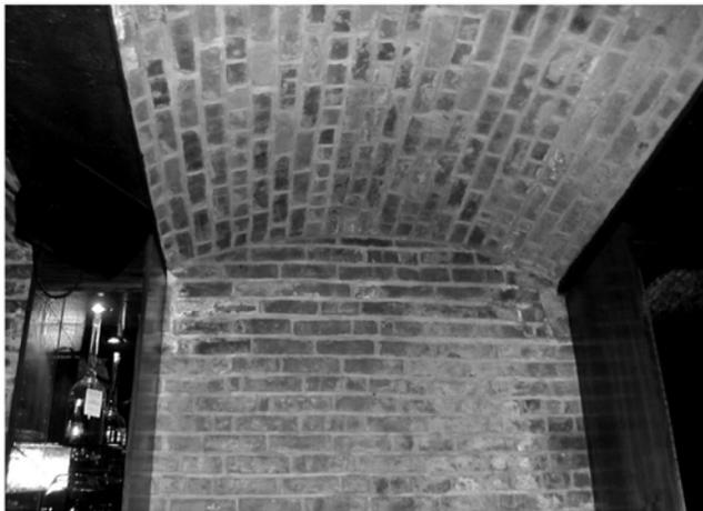
**12** Long view of the brick arch of the street vault now incorporated into the bar of the City Hall Restaurant on Duane Street. View is looking toward the brick street wall. Elements of the restaurant's downstairs bar are to the left. (Geismar 5/19/05)
