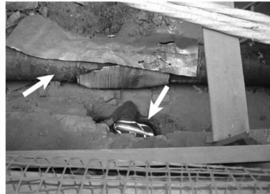
**e.** Excavator in the pit under excavation next to north wall (right arrow). A partially exposed steam pipe (left arrow) that runs down the center of the trench is next to the pit. The view is looking down from above the trench. (Geismar 5/9/05)
