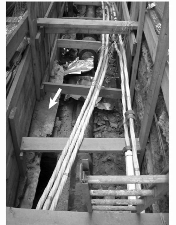
**h.** View of utility trench looking east from above. Note remnants of arched brick construction (arrow) above the north stone wall (not visible). (Geismar 5/10/05)
