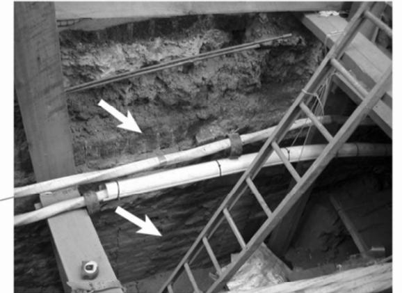
**g.** View of south wall from above. "Soldier" bricks (upper arrow) under fill are visible above encased live wires. A brick inset, apparently a sealed-off access, in the stone wall (lower arrow), is visible below the wires. (Geismar 5/10/05)
