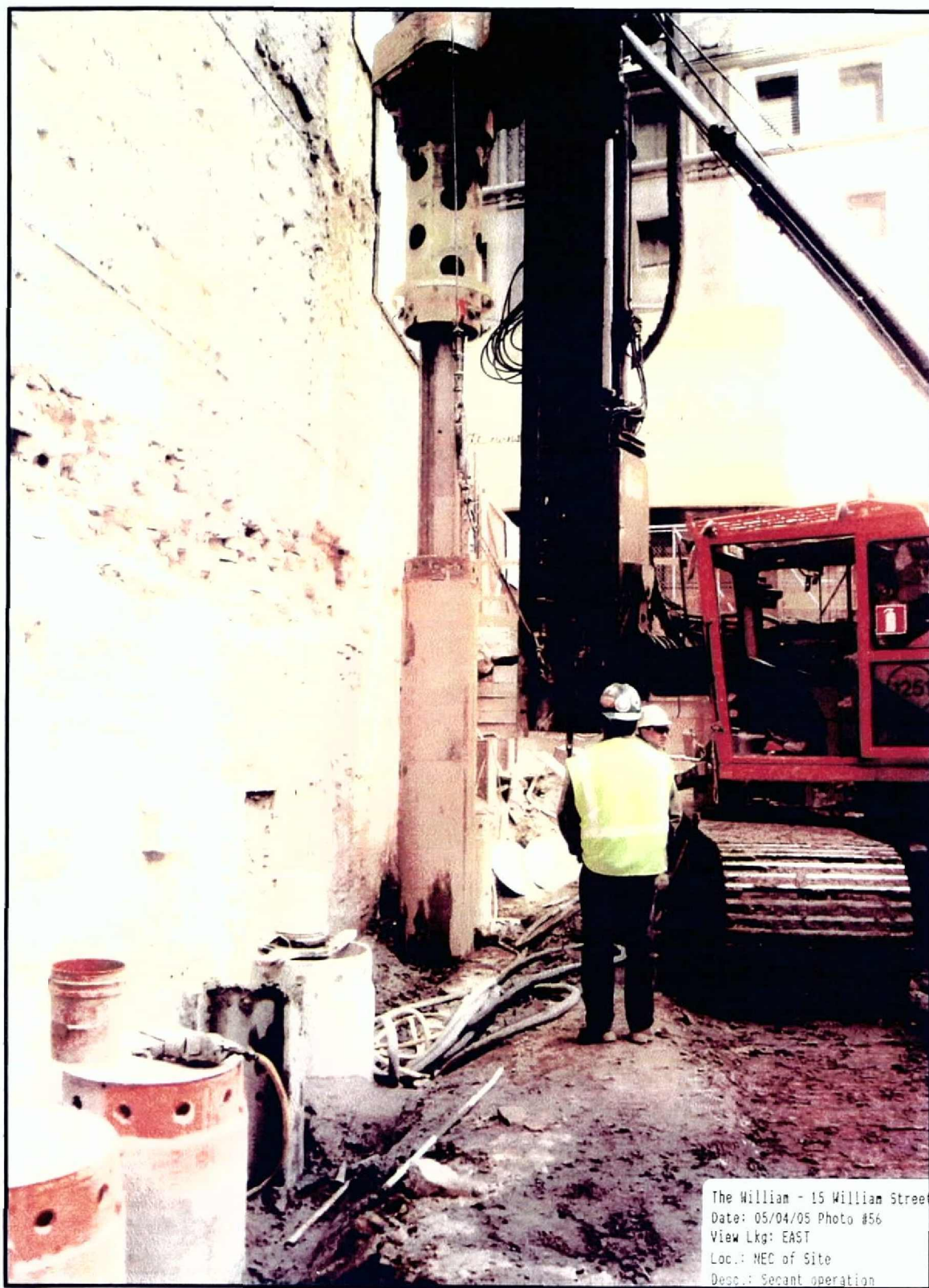
Photograph 7. Northeast Corner of Project Site looking towards the East. Secant Piles being driven along APE perimeter. (provided by Bovis Lend Lease)
