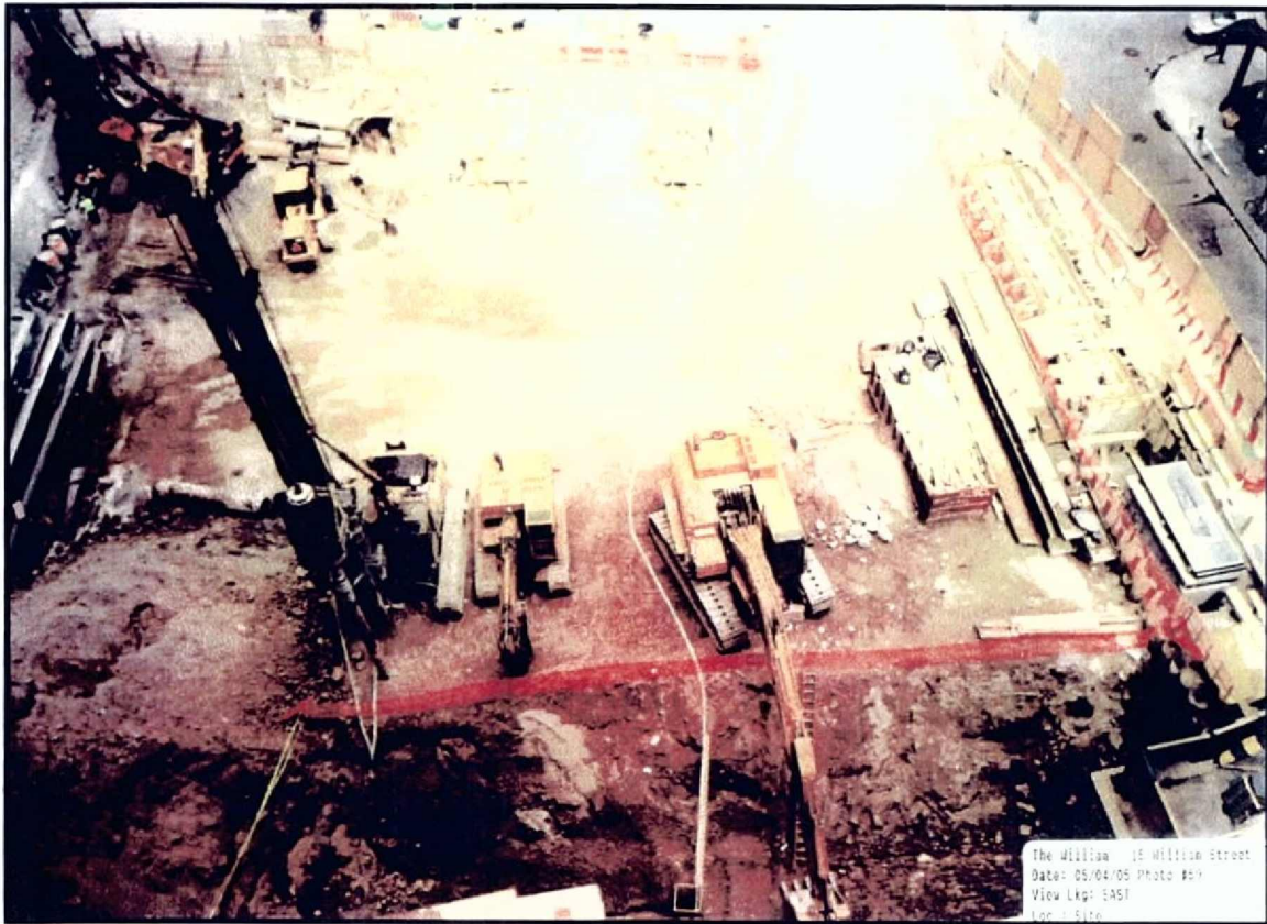
Photograph 5. Project Excavation for the relocation of steamline and for easement. (provided by Bovis Lend Lease)
