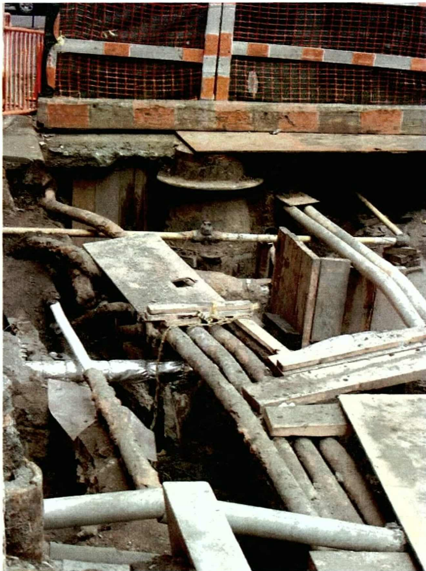
Photograph 18: Utility work in Platt Street within 20' of Pearl Street, immediately out of APE. Note the extensive network of underground utility pipes and structures, and the extent of excavation around them.
