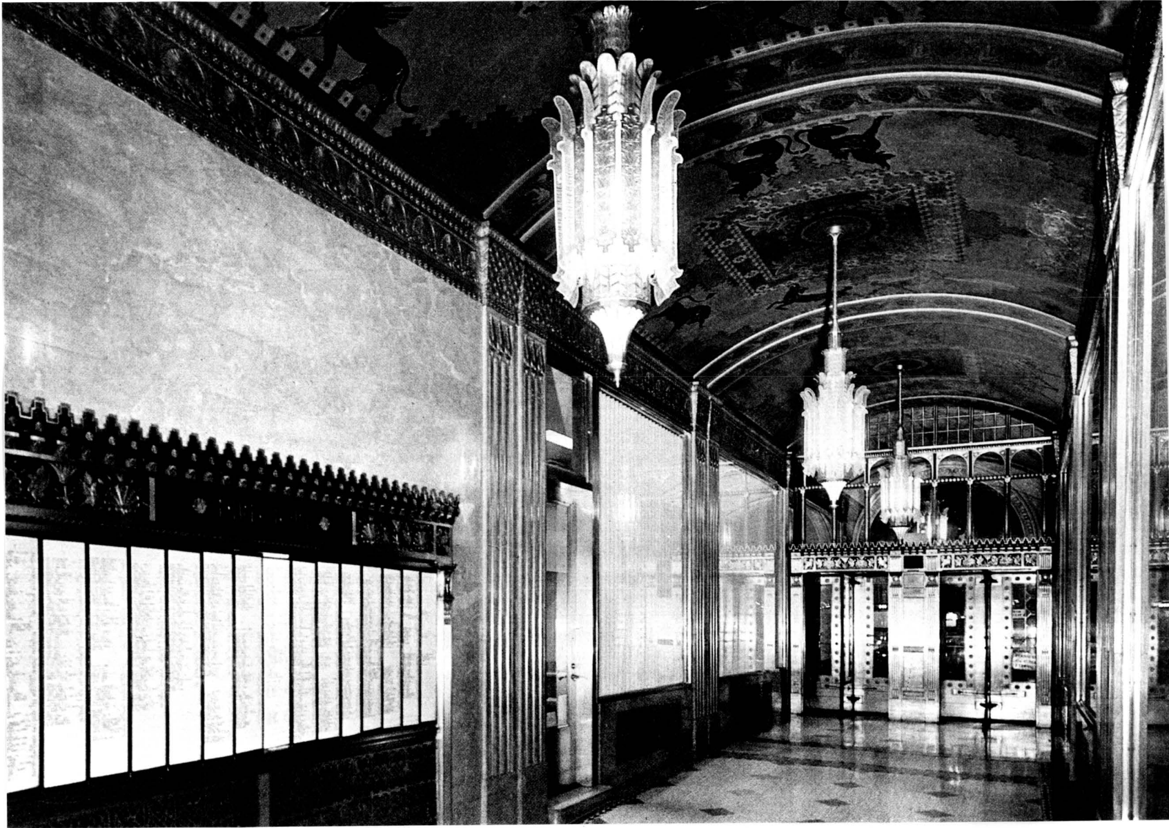
Detail: Fifth Avenue corridor, view to the southwest (toward Fifth Avenue).
