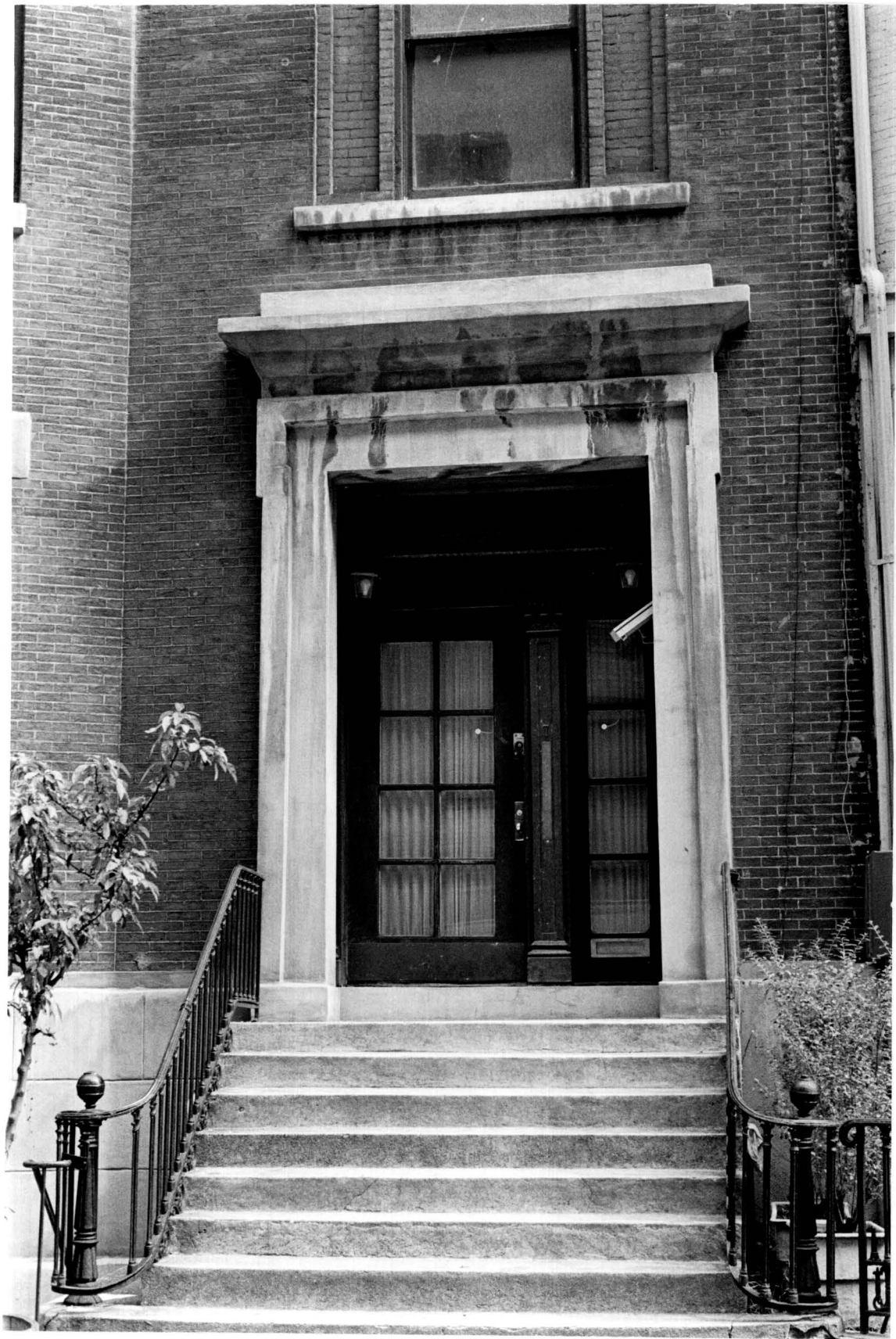
7 West 16th Street Building (entrance detail)
